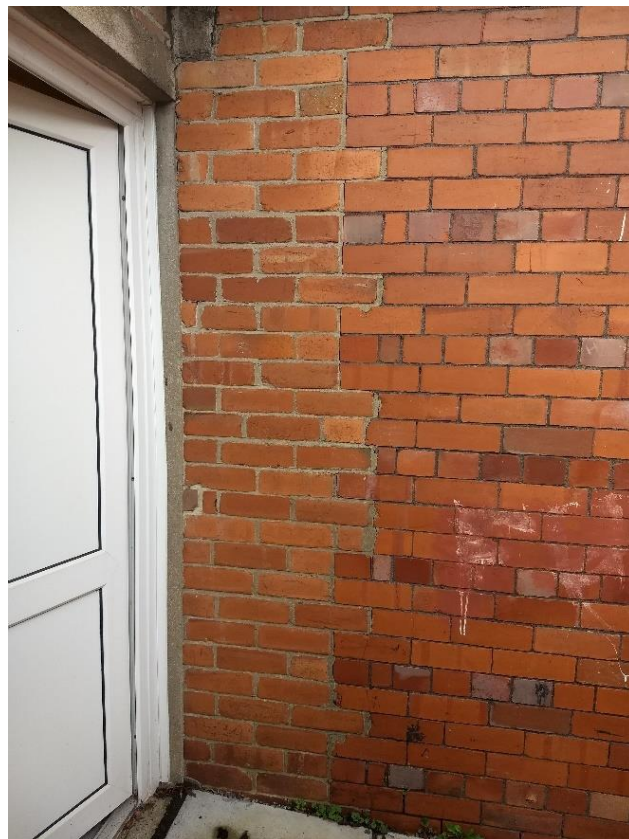
Photo 6 - Oldest Part 1 (right hand side) and later built Part 2 (left hand side) external masonry wall joined together with a key brick every three courses at the South East elevation
