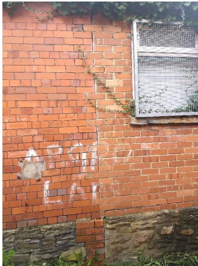
Photo 7 - Older Part 1 (left hand side) and later built Part 2 (right hand side) external masonry wall joined together with a key brick every three courses at the North West elevation
