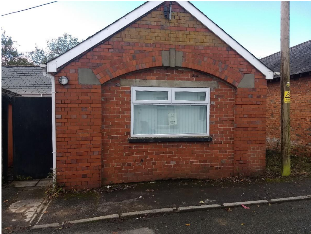
Photo 1 - North East front elevation of the building
