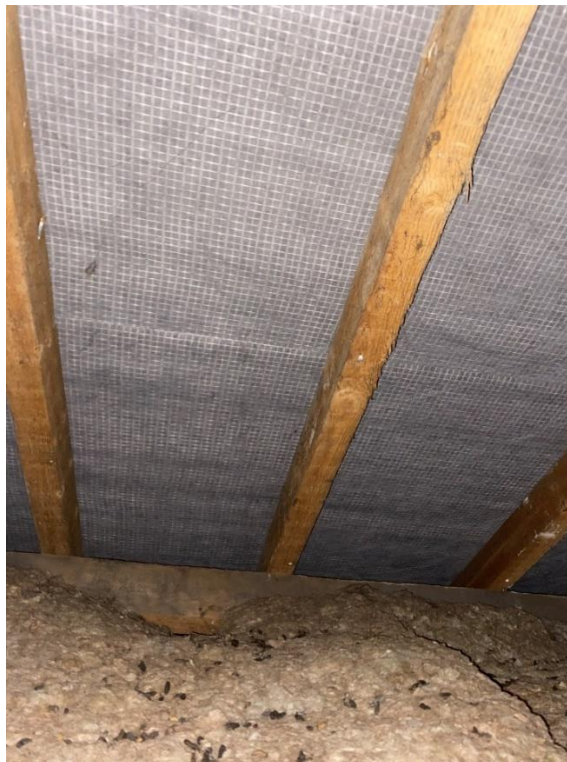
Photo 26 - Part of the roof showing rafters and the purlin close to ceiling level
