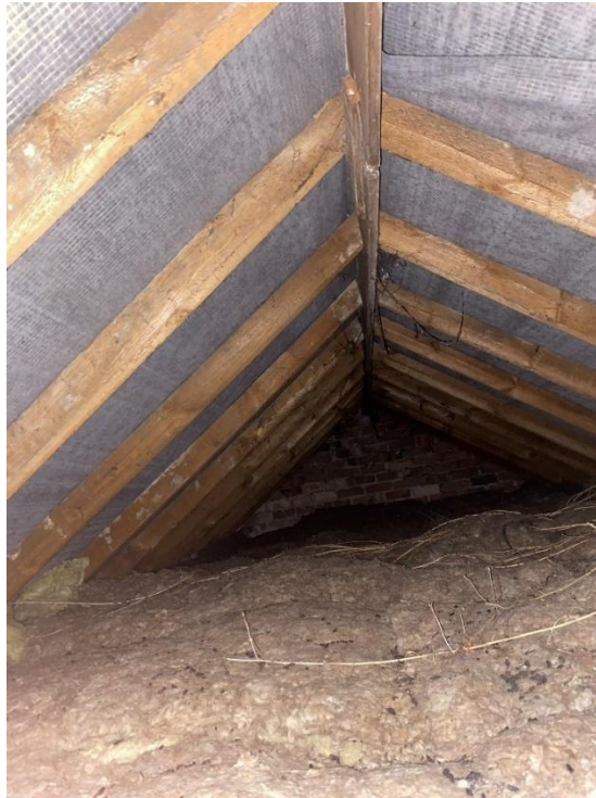
Photo 25 - The roof has been formed with cut rafters spanning from the ridge timber beam to the external walls
