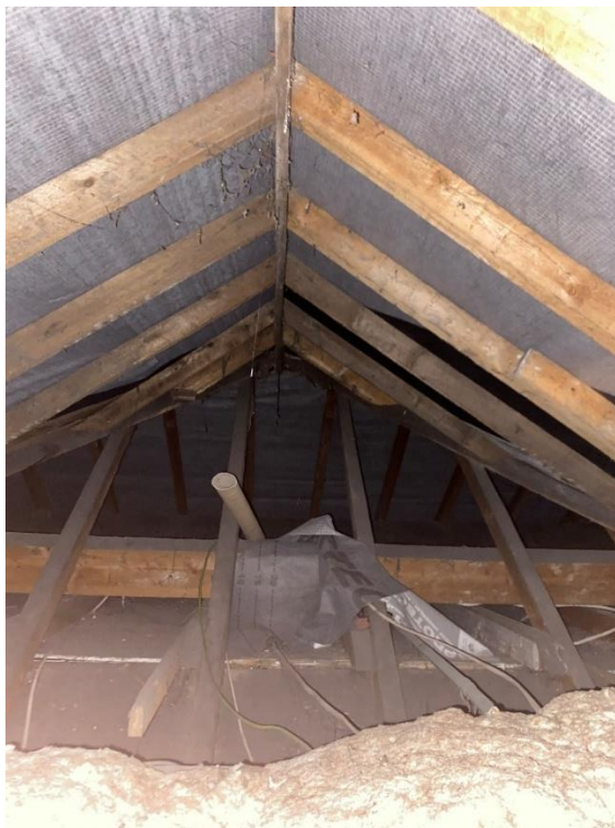
Photo 24 - Part of the roof, rafters and ceiling joists appear to be supported on the 300mm internal masonry wall
