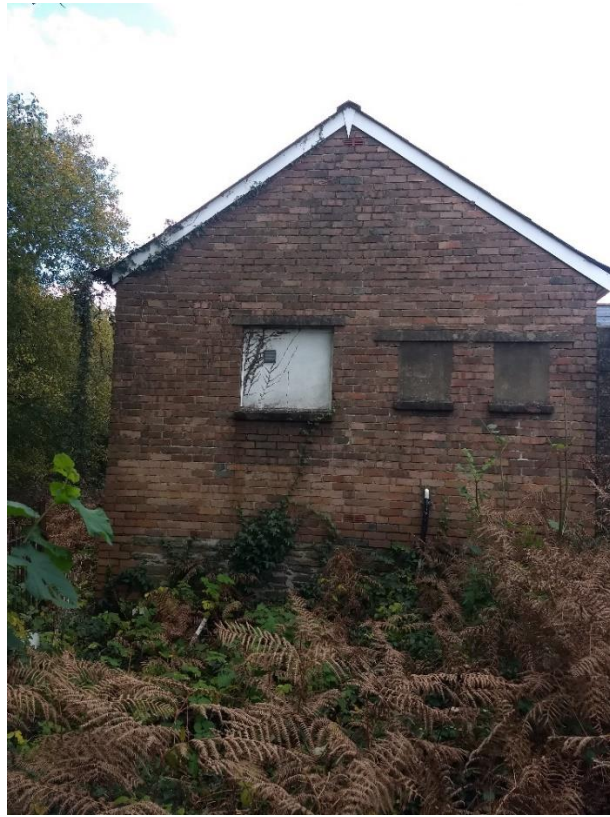
Photo 3 - Part of the South East left hand side elevation
