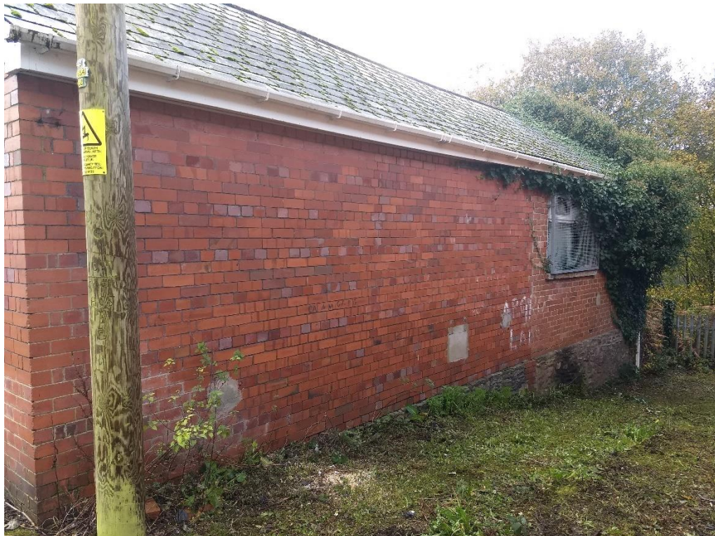
Photo 2 - North West right hand side elevation
