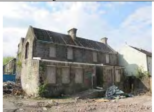
Northern elevation of building 1
