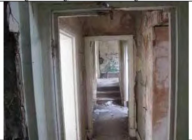
Interior of building 1
