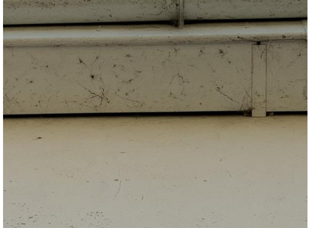
Photo 6: Gap behind uPVC soffit
