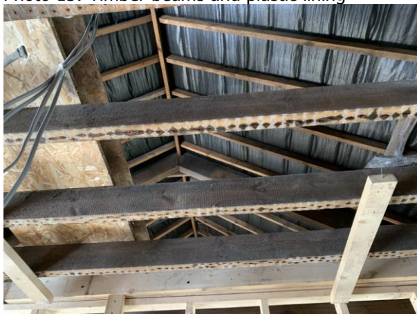
Photo 13: Timber beams and plastic lining
