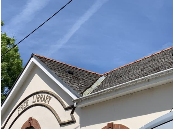
Photo 5: Roof tiles and lead flashing
