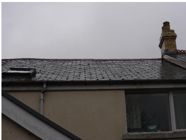
Figure 9 - Roof of terraced house
