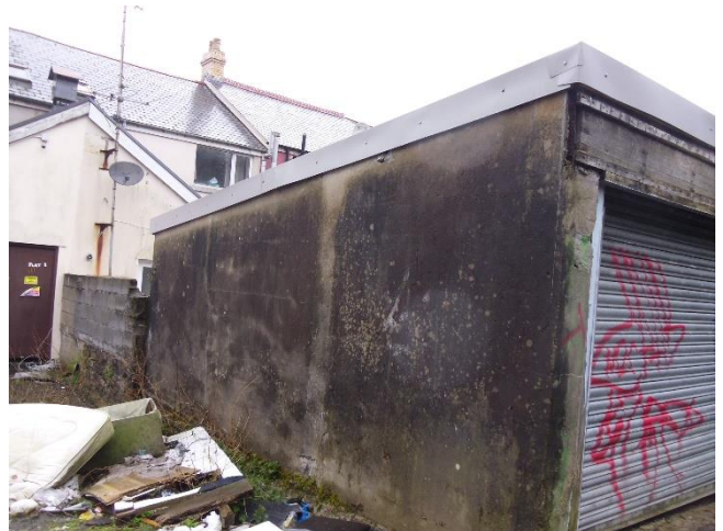
Figure 8 - Western aspect of the garage and roof of terraced property
