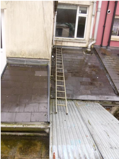
Figure 5 - Rear of terraced property
