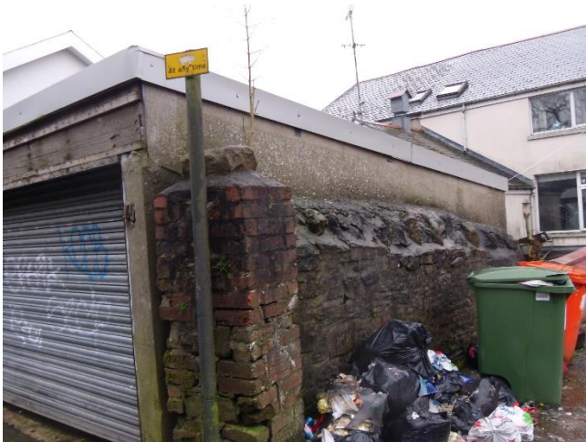
Figure 7 - Eastern aspect of garage and roof of terraced house
