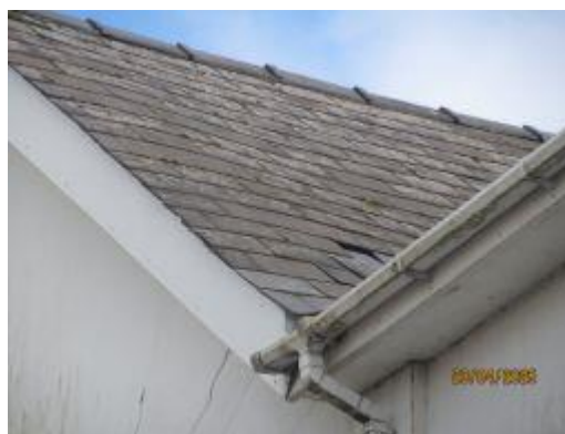
Missing slate providing access to a cavity between a layer of bitumen felt and slate.
