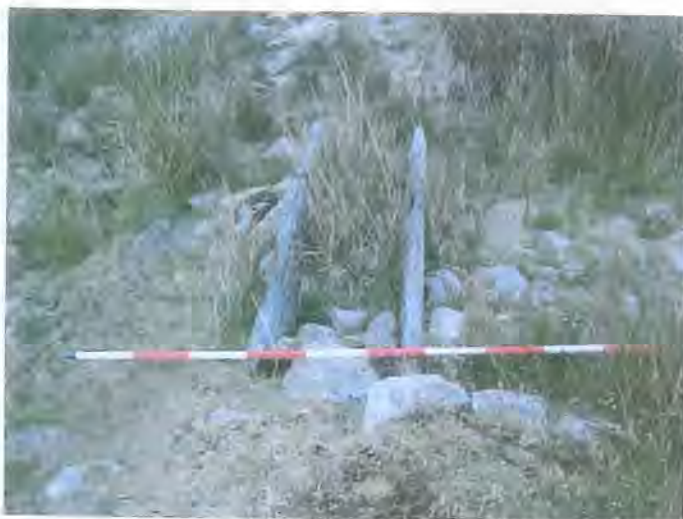
Plate 13: Stone-lined outfall sluice 88030 at NW corner of Pond 85525, looking W
