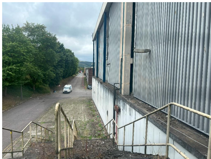
Photo 35: The external panelling is not flush to the wall and access is available throughout.
