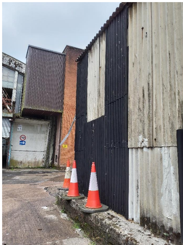
Photo 20: Example of the patched repair to building. There are gaps around many of the panels.
