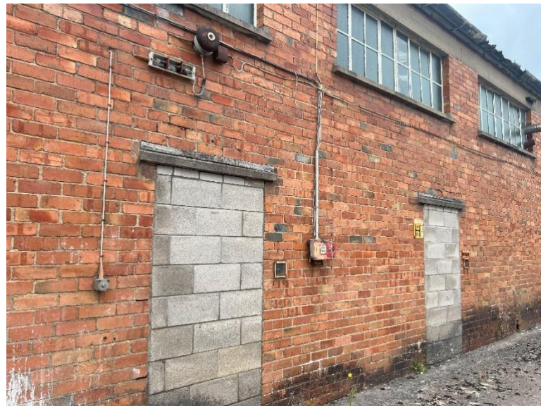
Photo 12: Shows how the building g has been closed for H&S reasons. The windows show the light levels from the roof lighting.
