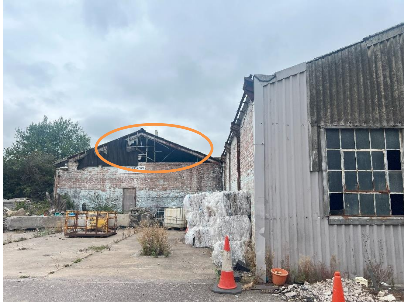
Photo 19: overview of building 5, the large open gable has been highlighted, and some broken windows are clearly visible.
