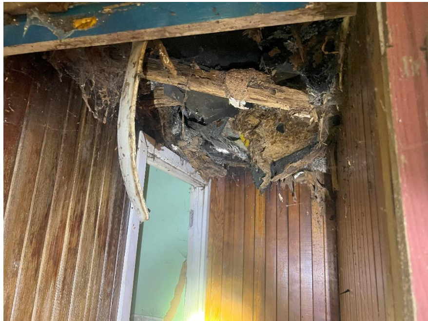
Photo 27: Example of the rot and damp within the roof.
