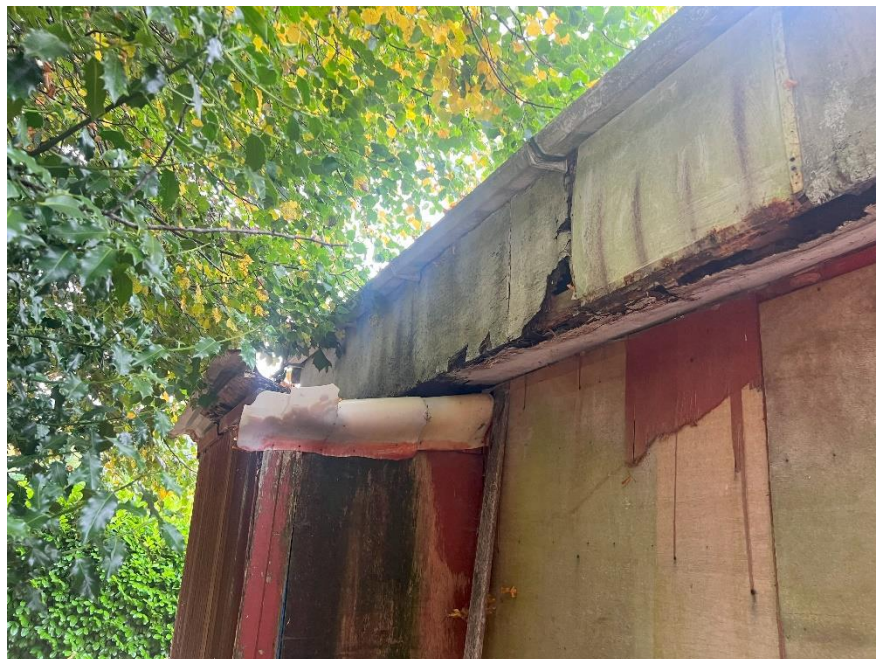
Photo 26: There is extensive damage to soffit boxes. Access is available for bats however it's likely the internal space is damp with little long term roosting potential.
