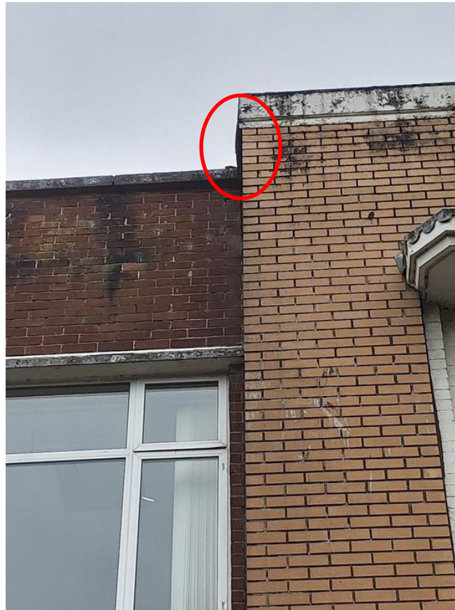
Photo 4: Lifting in roof felt
