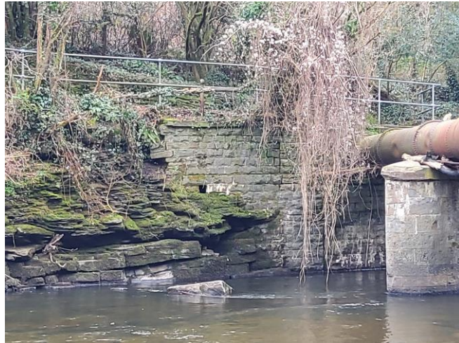
Photograph 5 Area of stone wall at south-east end of feeder pipe bridge. Gaps in walls suitable for bats to use for roosting.
