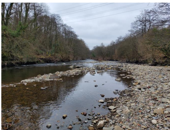
Photograph 2 View looking south downstream from feeder pipe bridge showing river and wooded banks.
