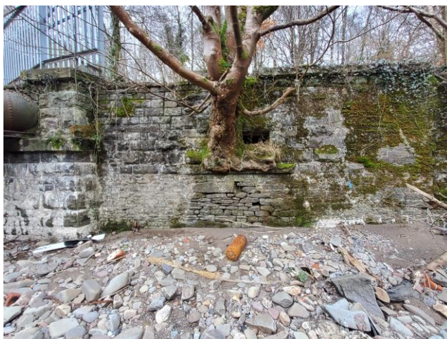
Photograph 4 Area of stone wall at north-west end of feeder pipe bridge. Gaps in walls suitable for bats to use for roosting.
