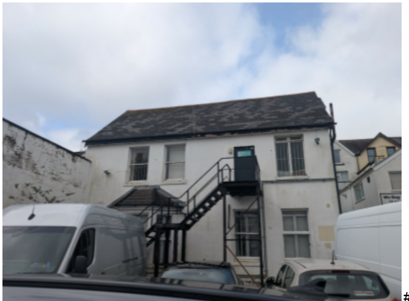
Plate 4- tight fitting slates
