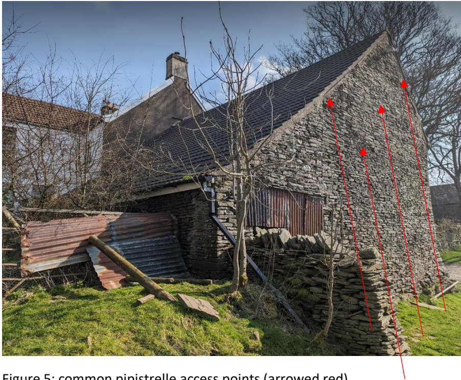
Figure 5: common pipistrelle access points (arrowed red)
