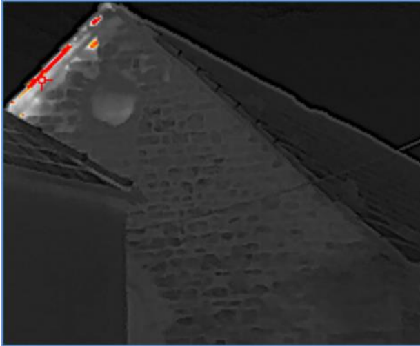
Photograph 17. View of eastern end of Building B.
