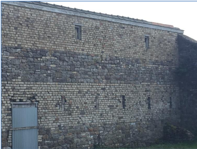
Photograph 15. Building C. The western elevation.
