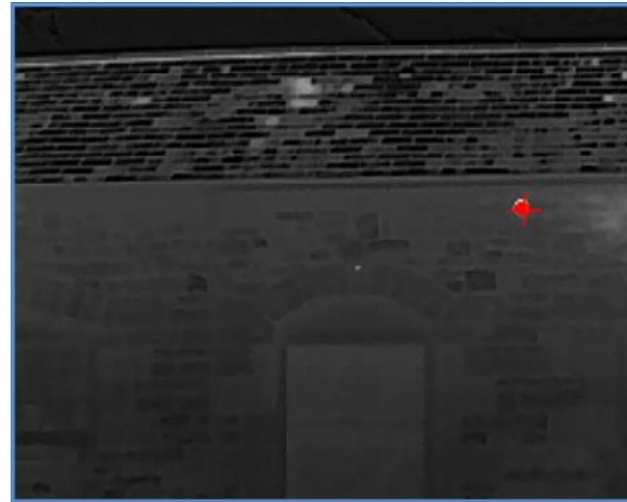
Photograph 18. View of southern part of Building B.
