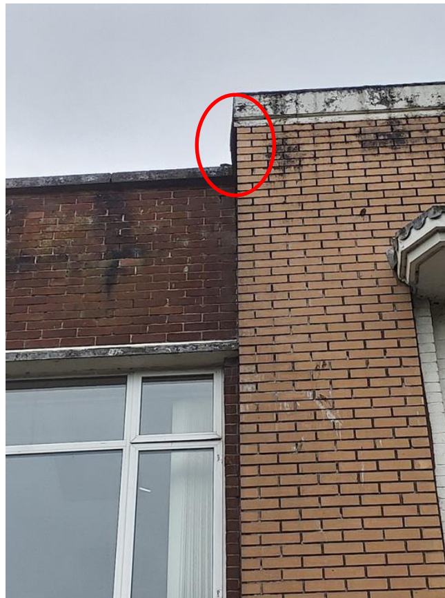
Photo 4: Lifting in roof felt
