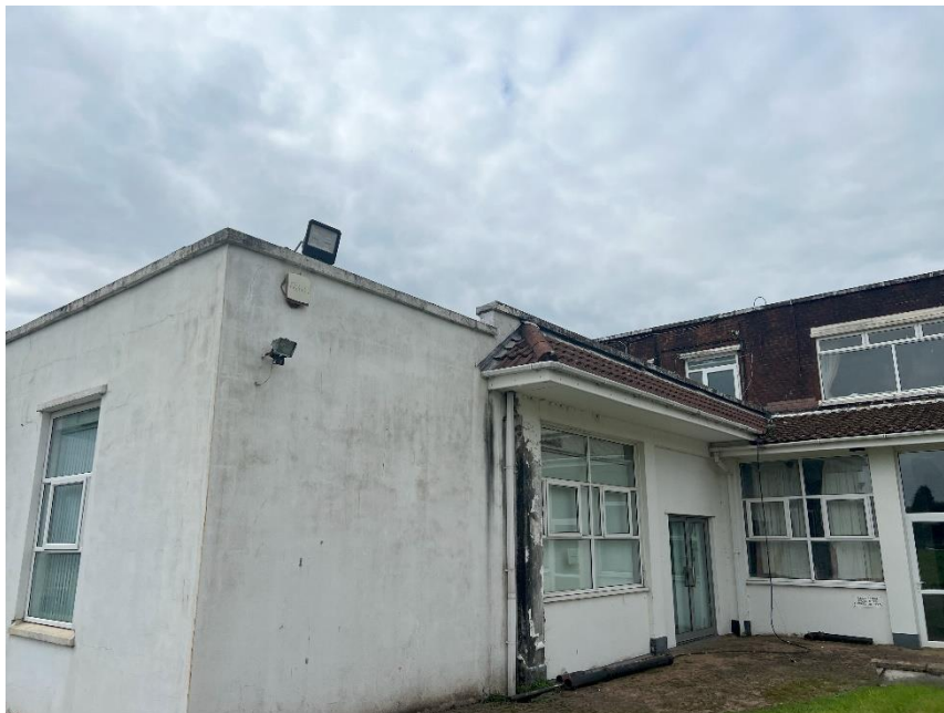
Photo 15: The flat roof is generally in good order with negligible PRFs, the small, pitched roof has lead flashing all around offering roosting opportunities.
