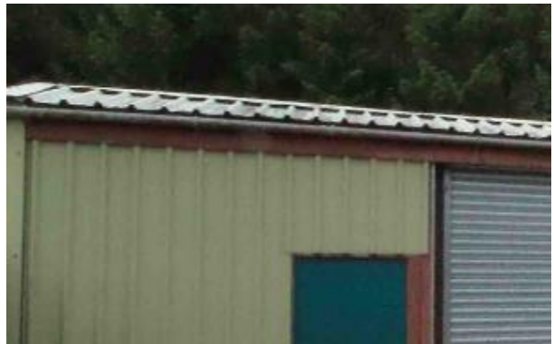
Photo 64: Wooden fascia boards providing voids
