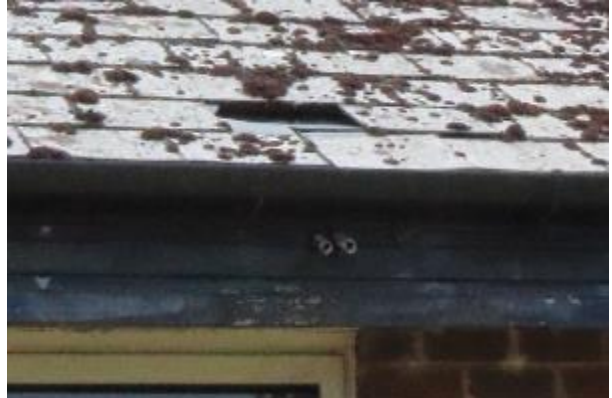
Photo 52: missing roof tile; north-east elevation
