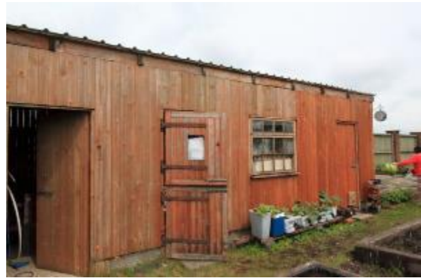
Photo 70: uncapped gable ends showing voids between roofing sheets and fascia boards; south-east elevation
