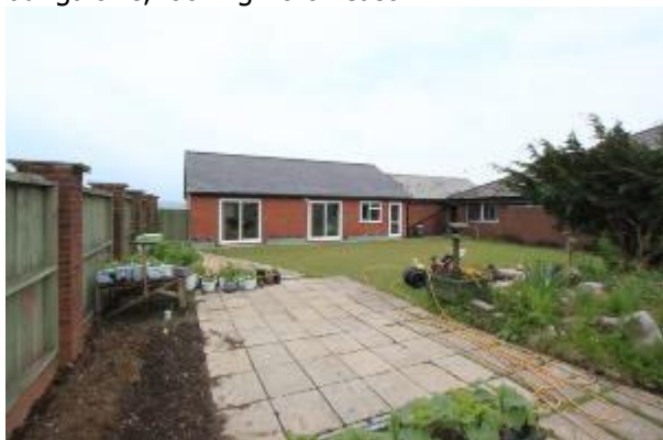
Photo 27: hardstanding to the rear of the staff bungalows, looking north-east
