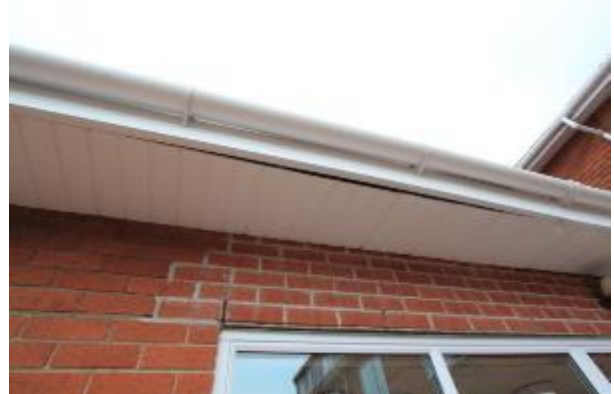
Photo 37: voids along soffit boards in the inner courtyard; north-west elevation
