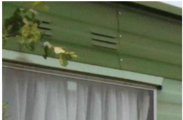
Photo 57: metal vents; south-west elevation
