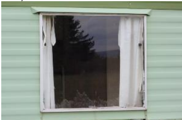
Photo 58: aluminium window typical of the static home; south-west elevation
