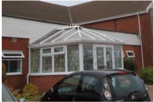
Photo 39: conservatory; south-east elevation
