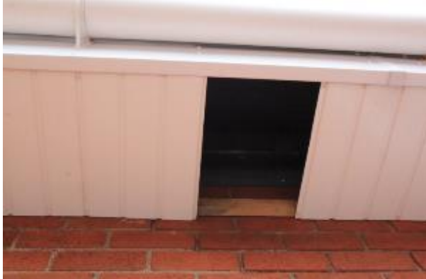
Photo 36: missing soffit boards in the inner courtyard; north-west elevation
