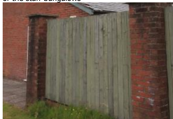
Photo 22: feather edge board fencing to the rear of the staff bungalows
