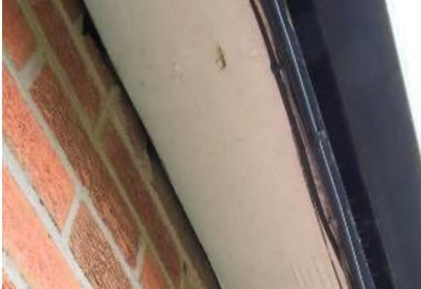
Photo 47: void in barge boards; south-east elevation
