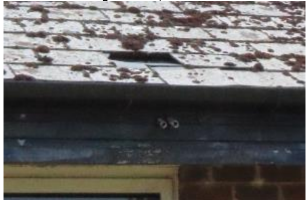
Photo 52: missing roof tile; north-east elevation
