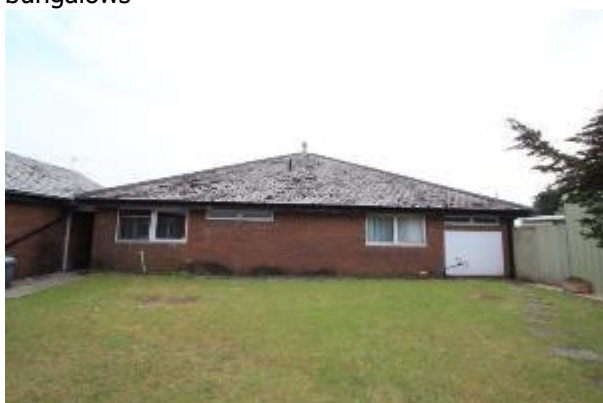
Photo 19: amenity grassland to the rear of the staff bungalows
