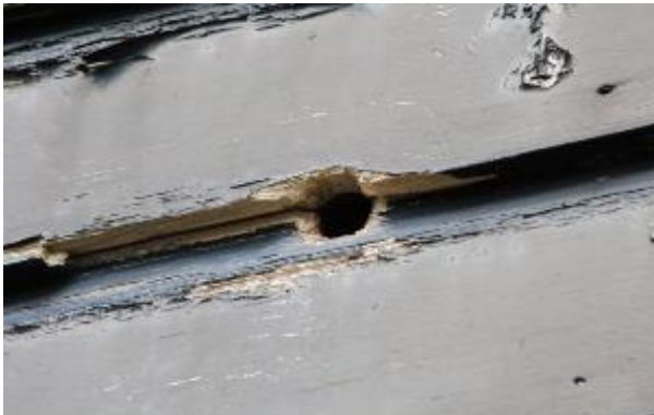
Photo 47: void in barge boards; south-east elevation
