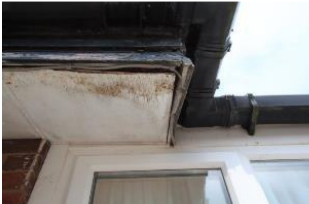
Photo 53: warped soffit boards; south-west elevation
