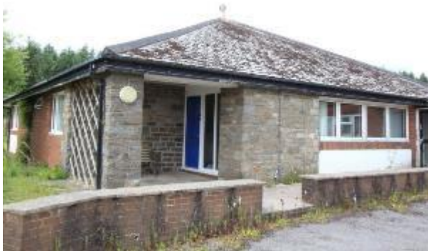
Photo 53: warped soffit boards; south-west elevation
