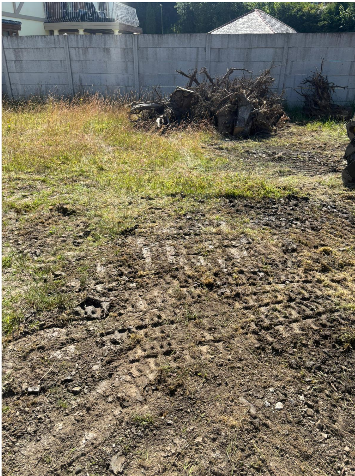
Figure 5 - Test pit 1 remediation
