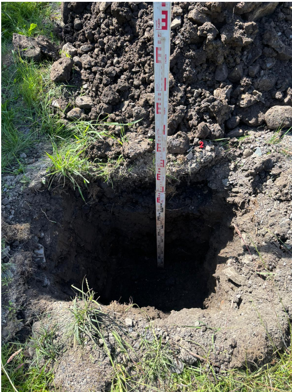
Figure 2 - Test pit 1 during excavation
