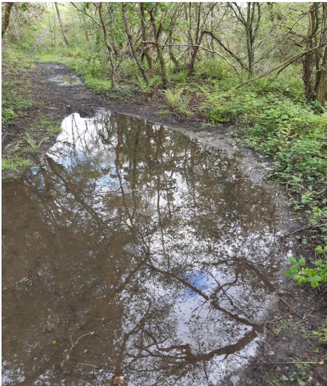
Plate 15 Stagnant water within the ‘Leat’ of the Cyfartha Tub Boat Canal and water found to be seeping from the leat and into the ‘hollow’ -12
