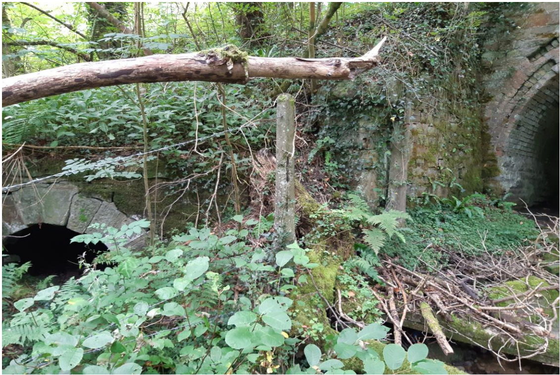
Plate 33 Photo showing a small culvert emerging adjacent to a much larger culvert beneath a railway line - 25
