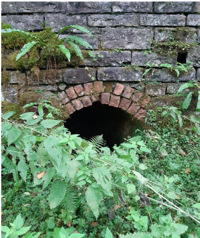
Plate 30 Photo of a brick lined culvert entrance within the base of the stone masonry wall of Cwm Pit - 23
