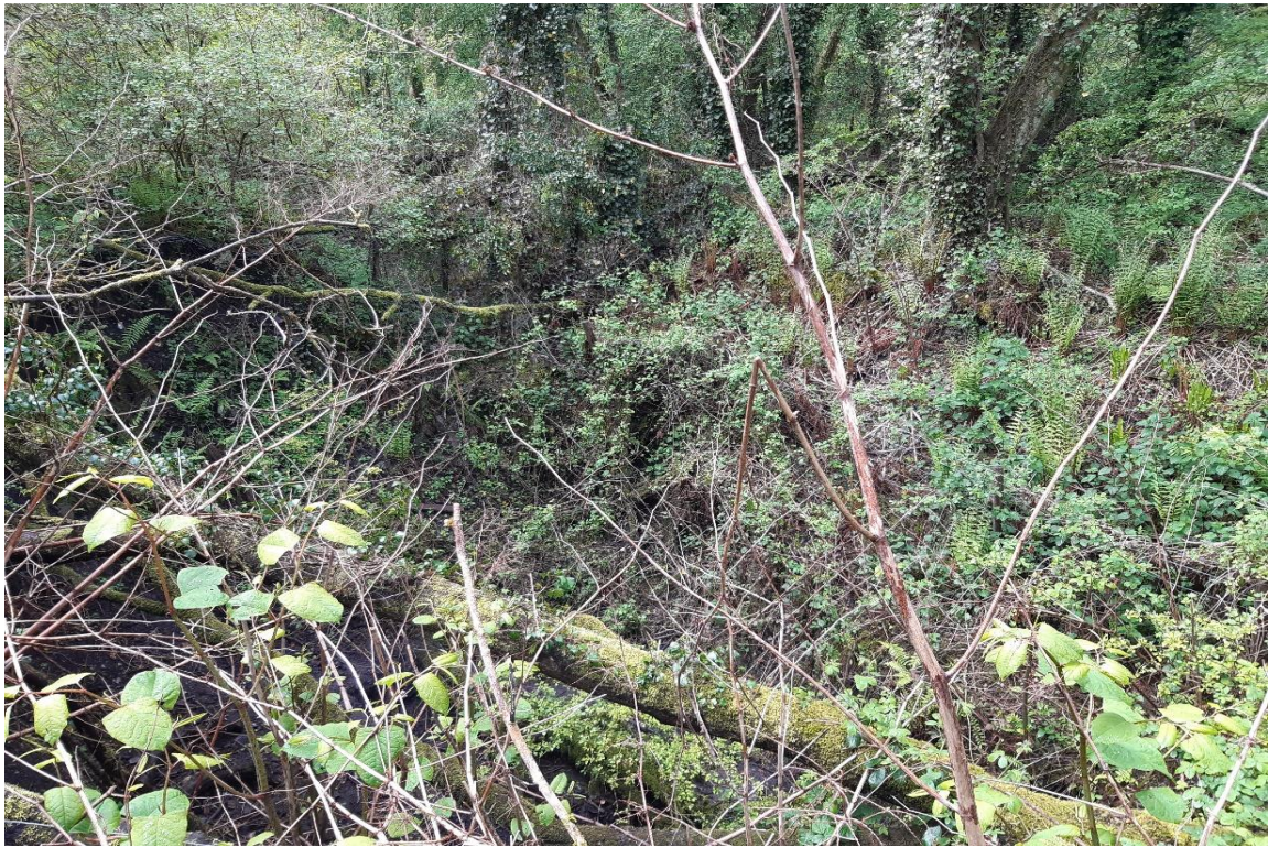
Plate 37 Photo viewing a large area of collapse which was dry at the time of the visit - 30
