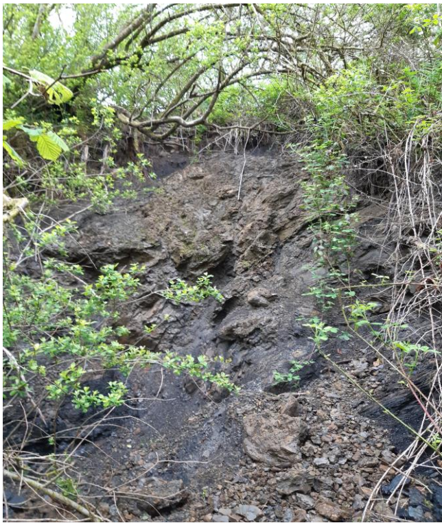
Plate 10 Photo showing exposed coal seam within cutting of the railway line. - 8
