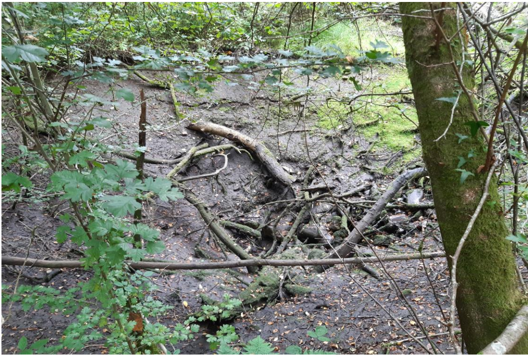
Plate 35 Photo showing an area of collapse - 27
