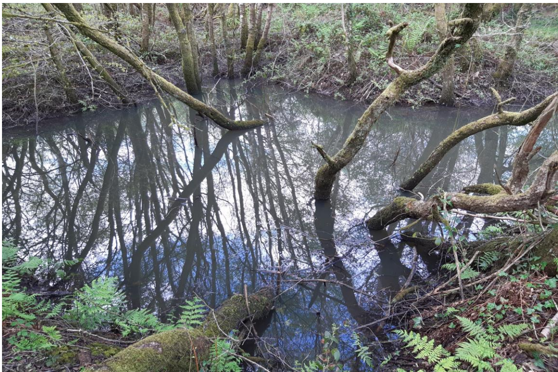
Plate 16 Stagnant water within the ‘Leat’ of the Cyfartha Tub Boat Canal and water found to be seeping from the leat and into the ‘hollow’ -12
