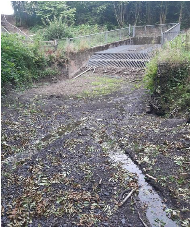
Plate 25 Photo of the Nant Cannaid culvert beneath the former Aberdare to Merthyr railway line - 18
