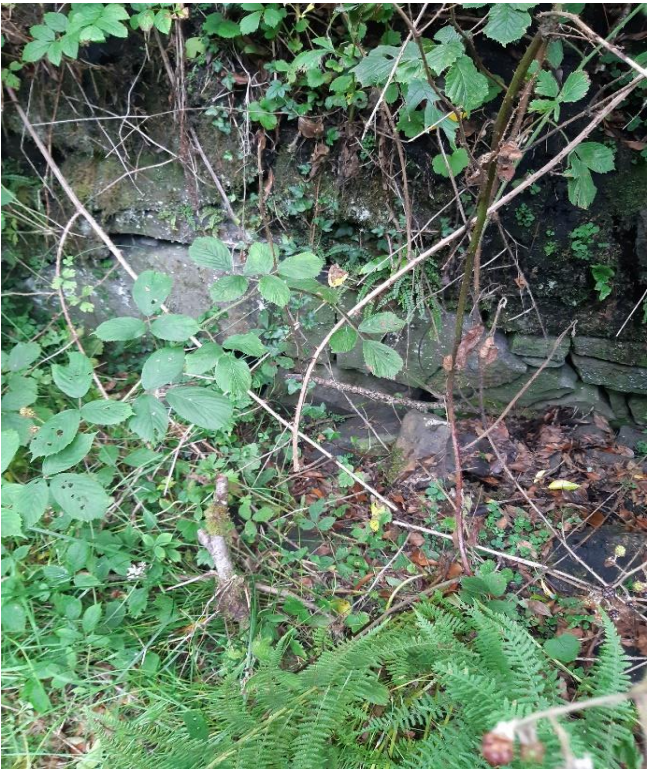
Plate 28 Photo showing a buried culvert outfall point on the bend of the Nant Cannaid prior to the culvert beneath the former Aberdare to Merthyr railway line. - 21
