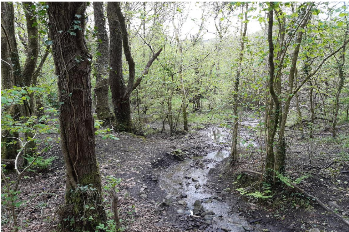
Plate 18 Water draining away from a break in the ‘Leat’ and discharging into the ‘hollow’ - 13
