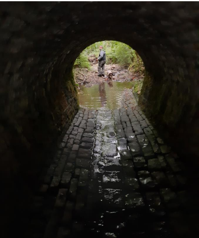
Plate 27 Photo showing the culvert for the Nant Cannaid beneath track crossing - 20
