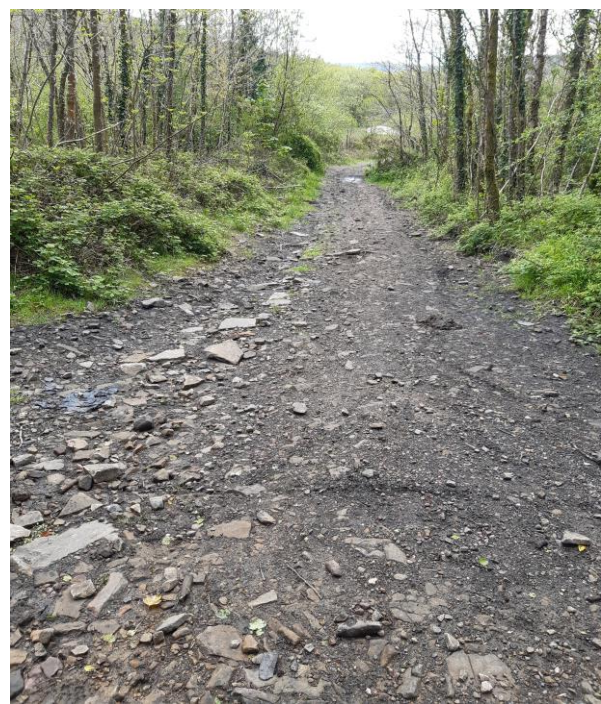
Plate 5 Photo looking eastwards along vehicle access track at damage which is the result of flood water overtopping from the ‘hollow’. - 4
