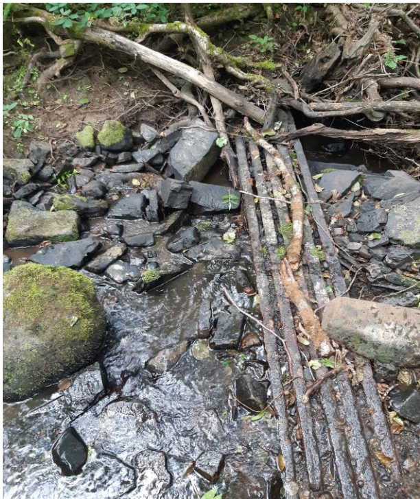
Plate 29 Photo showing metal tram lines within the bed of the Nant Canaid Stream - 22
