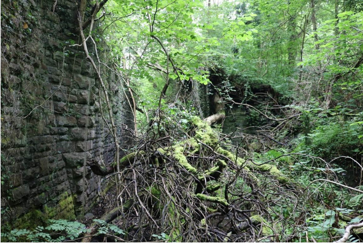
Image EDP 65: Former bridge across tramway at the Cyfarthfa Crossing.
