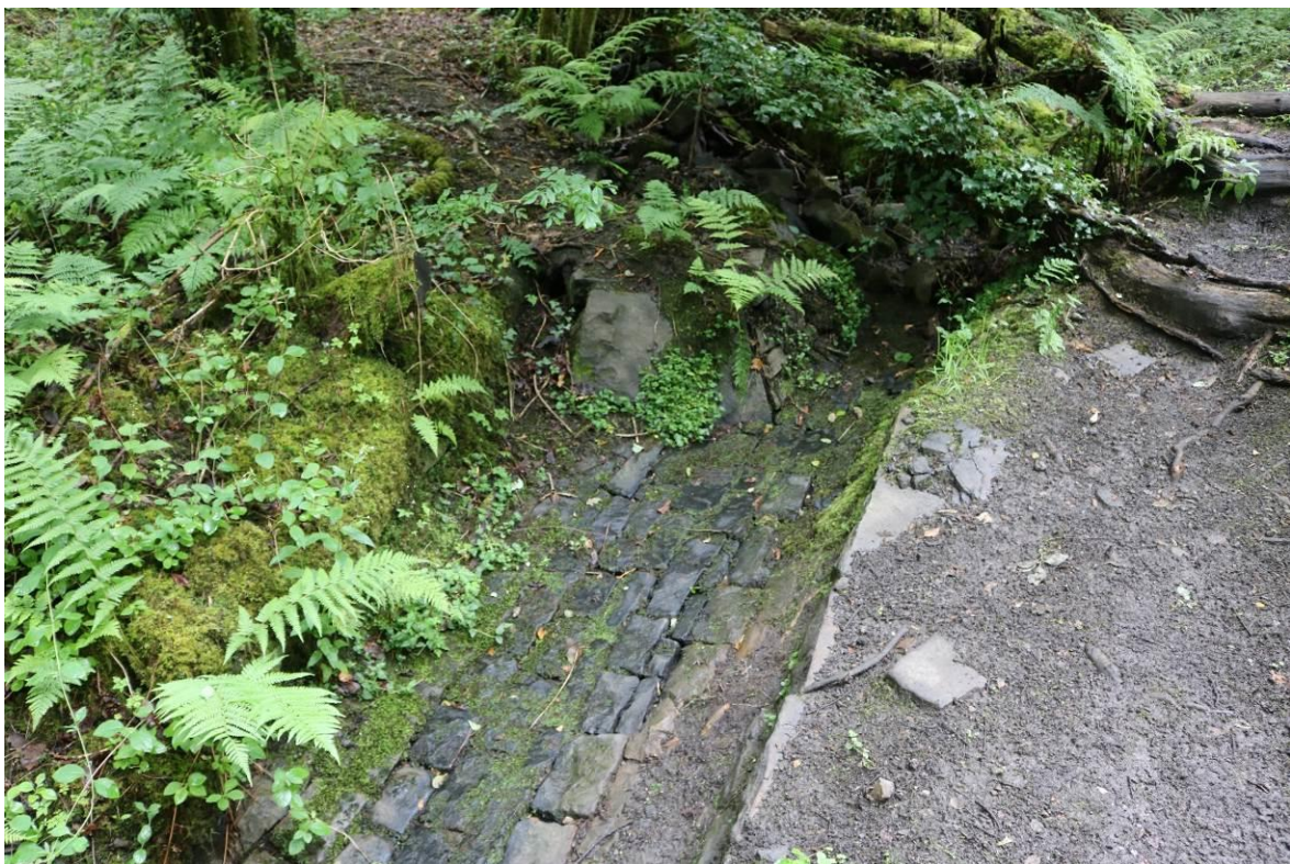
Image EDP 60: Stone lined culvert on the Vale of Neath Railway.
