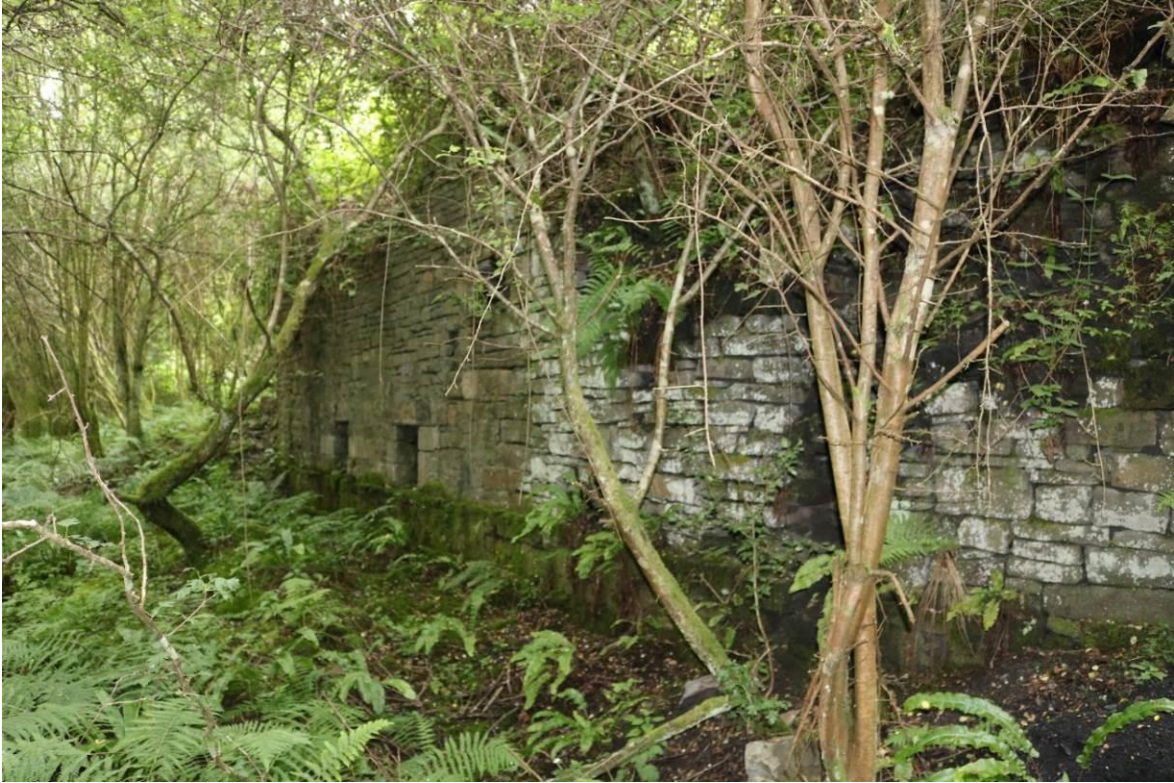
Image EDP 55: Possible loading bay building north of Lower Collier's Row.
