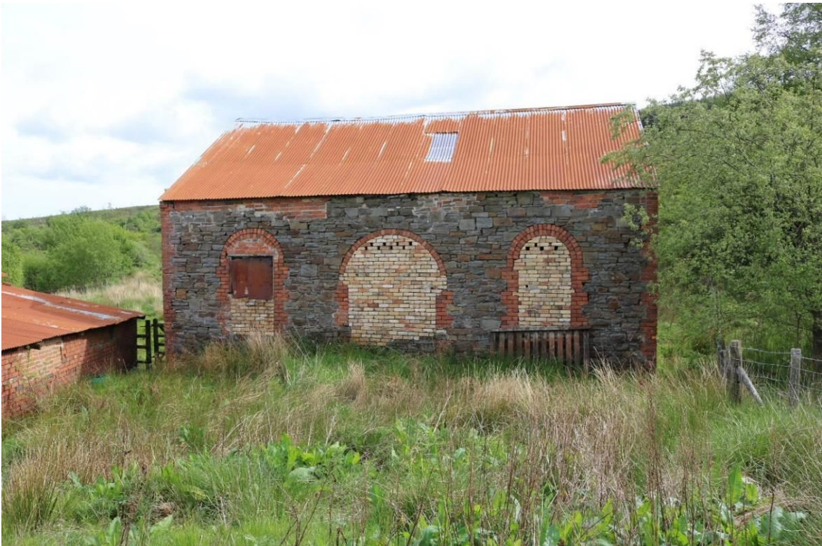
Image EDP 50: Probable engine house at the former Cwm Du Drift mine.
