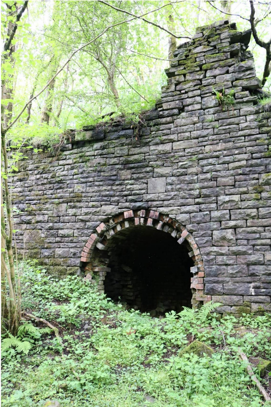
Image EDP 8: Furnace entrance at Cwm Pit.
