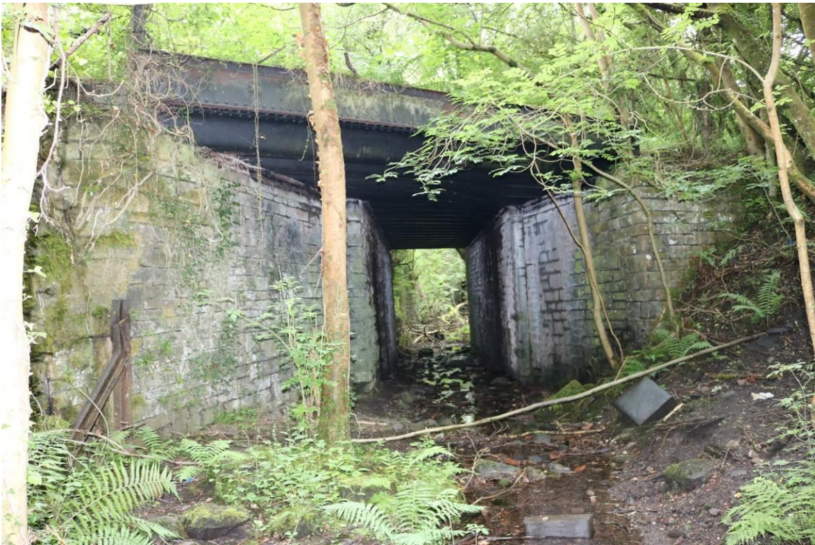
Image EDP 64: Iron bridge at the Cyfarthfa Crossing.
