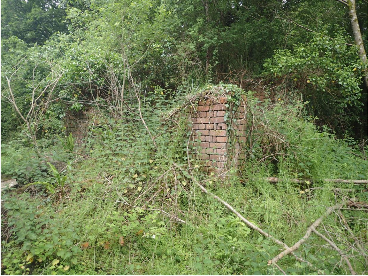
Image EDP 69: Brick structure revealed by vegetation clearance adjacent to the former Ynys Fach railway.
