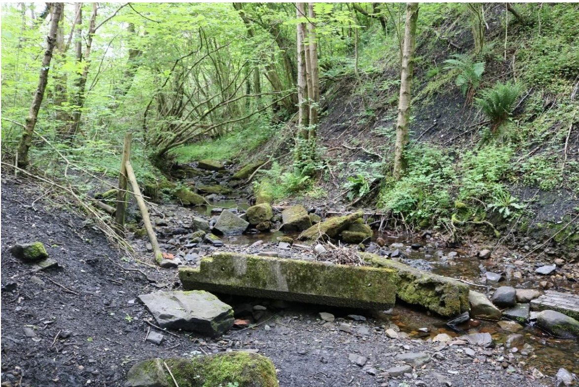
Image EDP 66: Rubble and concrete remains in the location of the former Cwm Pit Railway bridge across the Nant Cwm Glo.
