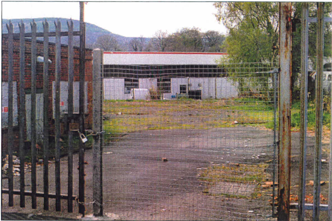
Plate 7: View looking westwards into Area F from access road
