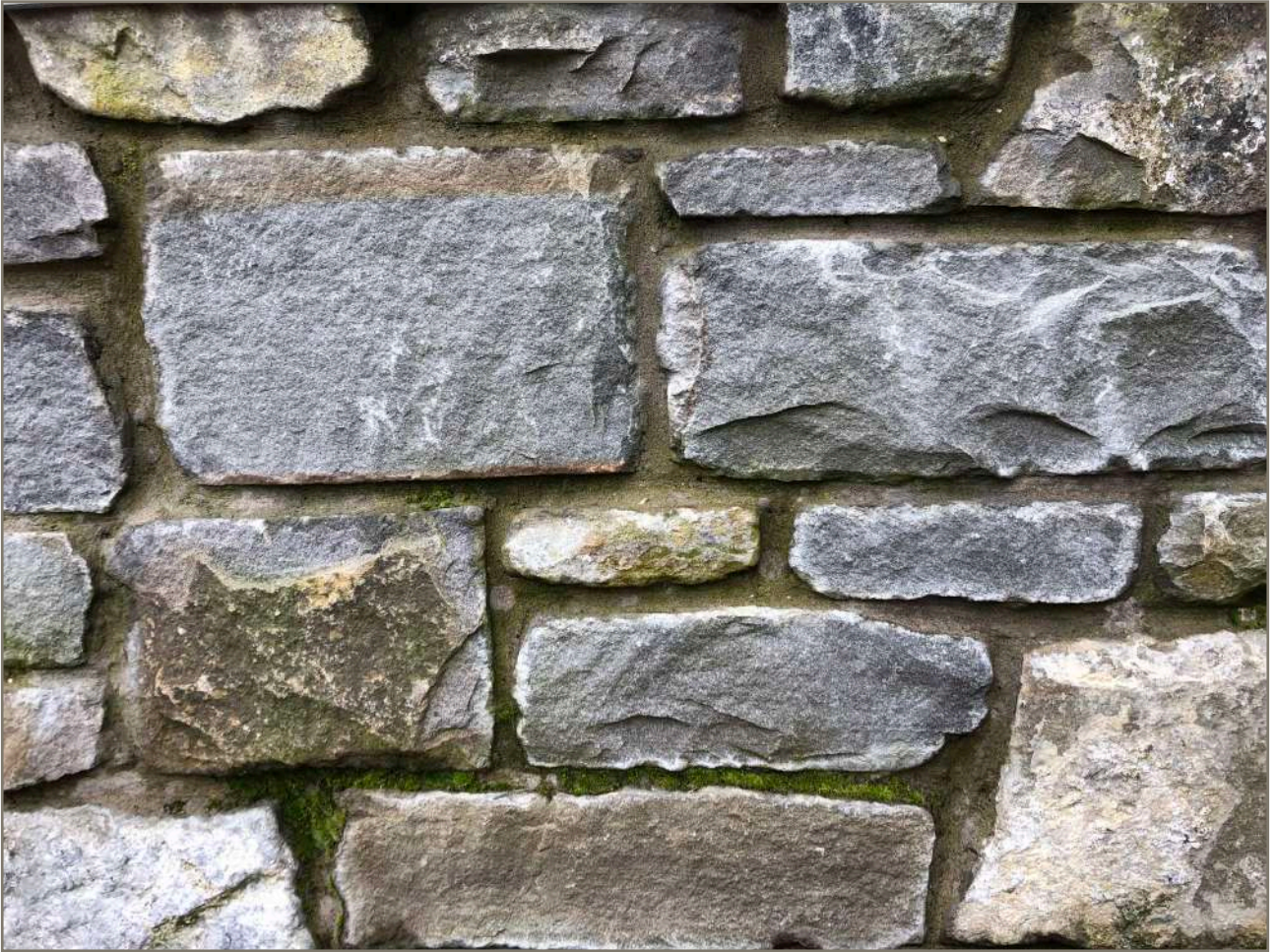
Image - Photograph of stone work to be used on dwelling. Re-used and reclaimed stone Pennant Sandstone throughout.
