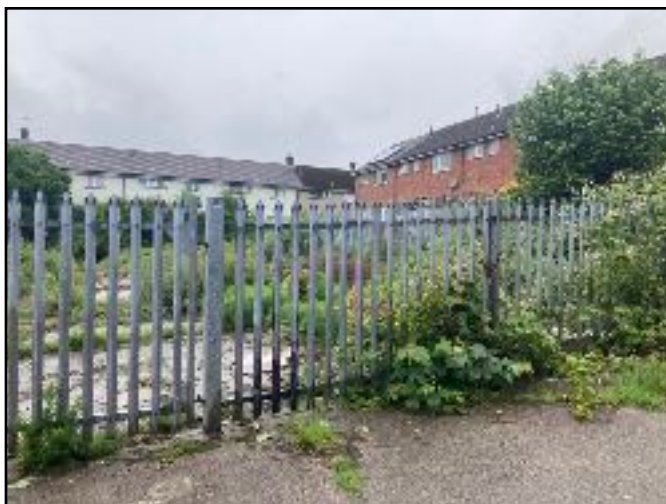
Photo.6. Looking into site through eastern boundary
