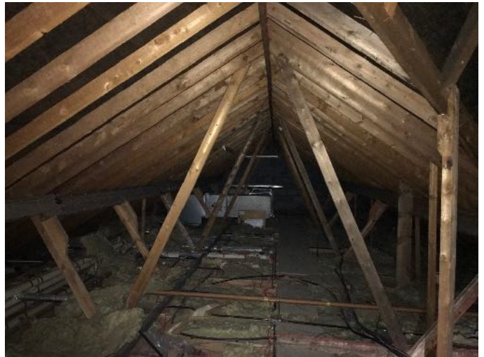
View of internal attic space
