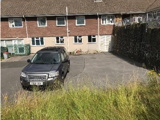
Tarmac hardstanding to east of building
