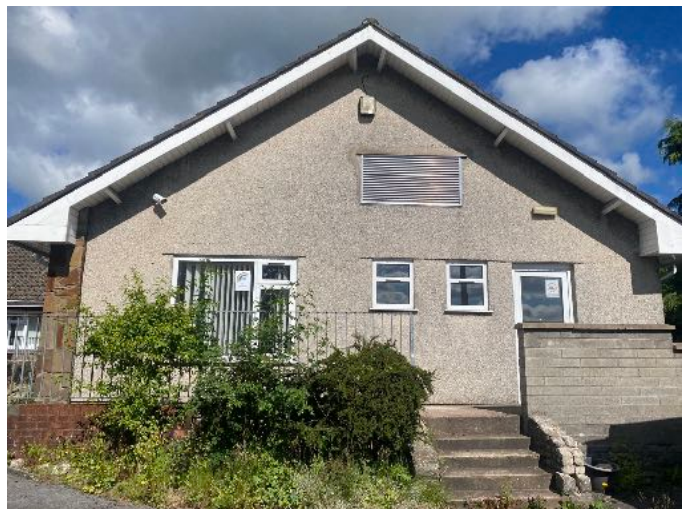
East gable end
