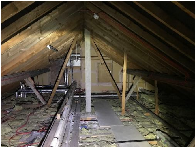
View of internal attic space
