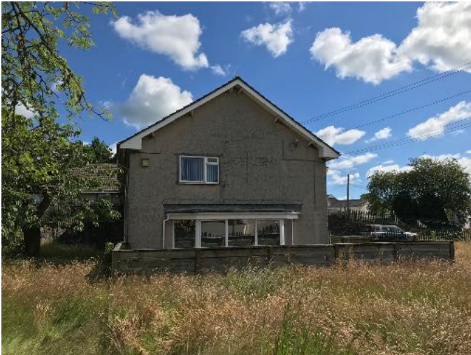
South gable end of building
