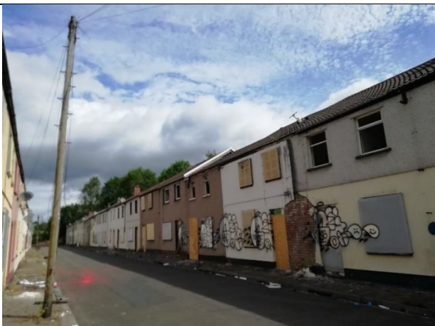
Figure 10 – View along Taff Street to north
