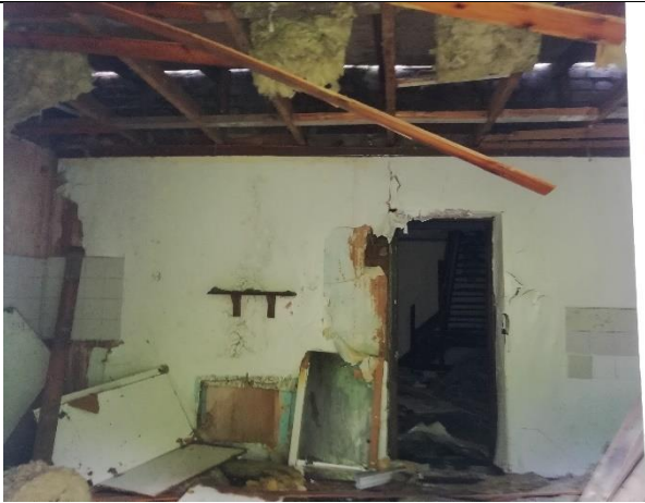
Figure 12 – Interior view (from outside) of south-westernmost property
