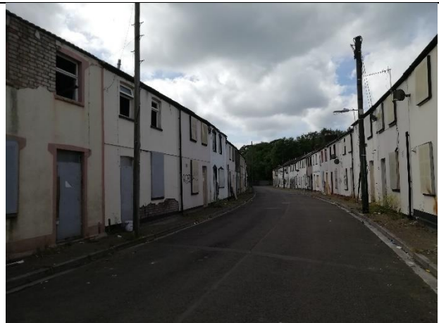
Figure 17 – View to south along Crescent Street.
