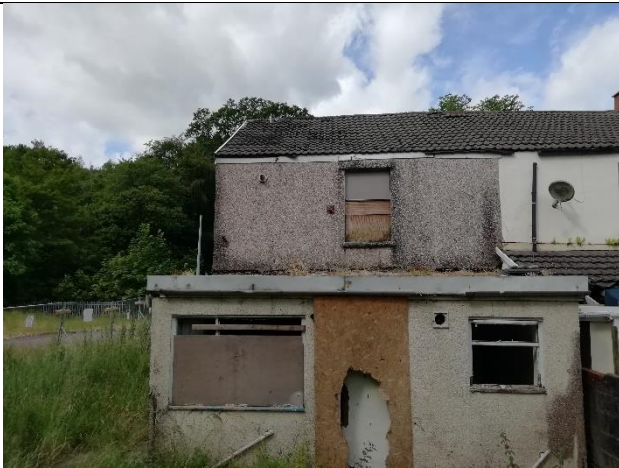
Figure 6 – Typically open property at south-eastern end of Taff Street (roosts at ridge as well as shown in Figure 6)
