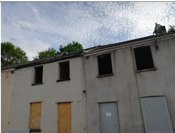
Figure 14 – View of open windows along Taff Street
