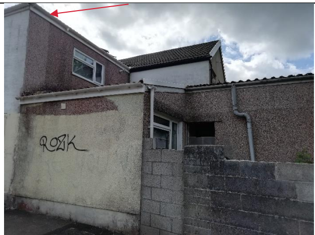
Figure 15 – North-westernmost property with common pipistrelle roost (at roof light)
