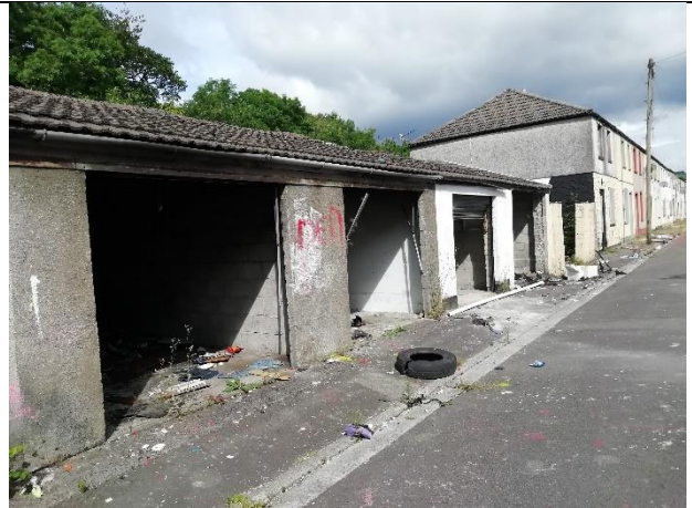
Figure 9 – Garages on Taff Street
