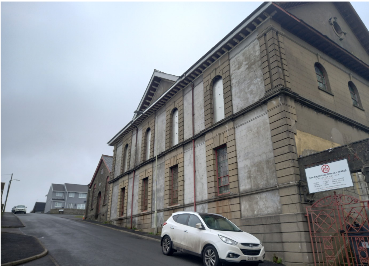
Image EDP A1.11: View of Grade II listed building Bethania Independent Chapel, illustrating its appearance.
