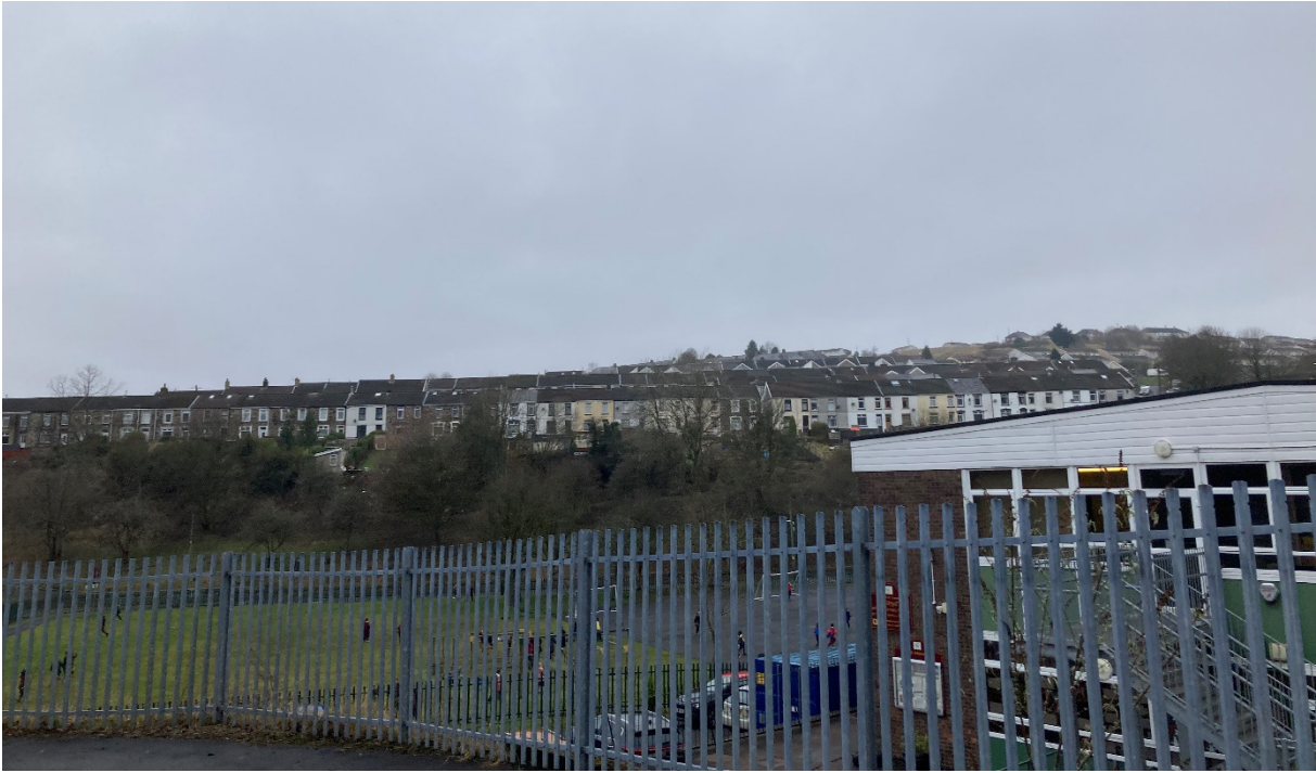
Image EDP A1.14: View south-west to terraced housing set in various patterns within the Gurnos and Galon Uchaf Historic Landscape Area, illustrating the urban character of HLCA 050.
