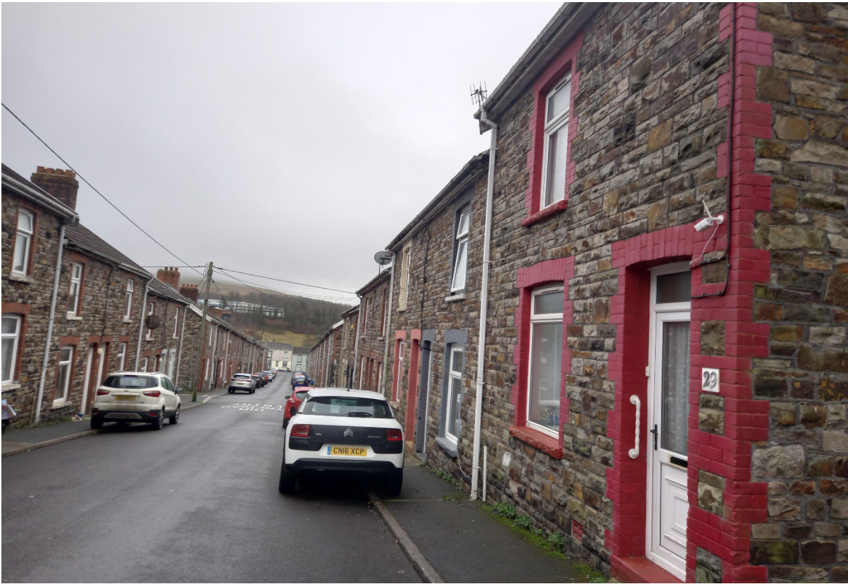
Image EDP A1.12: View south-east of Urban Street, illustrating the frontages of the houses, which is an aspect of the special architectural character of the Council and Urban Street Conservation Area.
