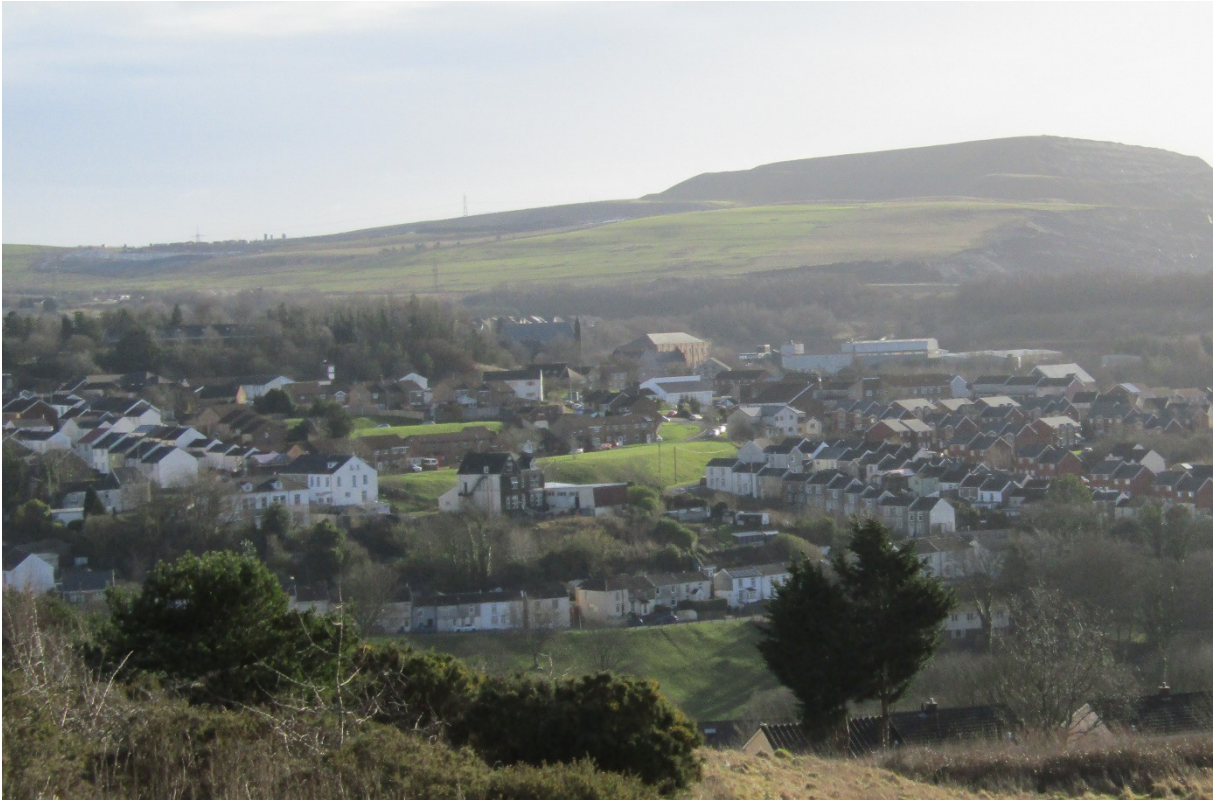
Image EDP A1.4: View east from the site towards the listed buildings within Dowlais, illustrating glimpsed, partly obscured views towards the Grade II* listed Dowlais Engine House, Grade II St Johns Church and Grade II Bethania Independent Chapel, although within the context of the wider built settlement, and at such a distance to not allow for appreciation of the buildings.
