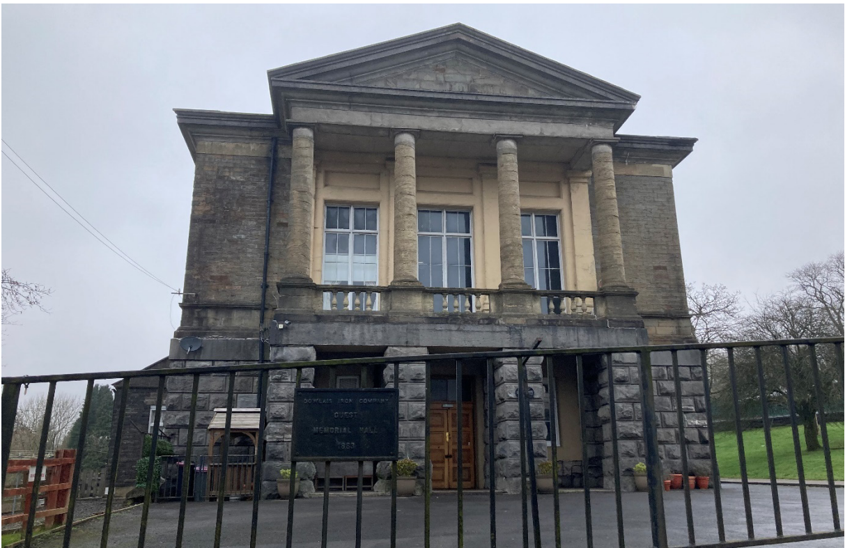
Image EDP A1.13: View of the Grade II* listed Guest Memorial Library, illustrating its striking architecture which makes a contribution to the special architectural character of the Dowlais Conservation Area.
