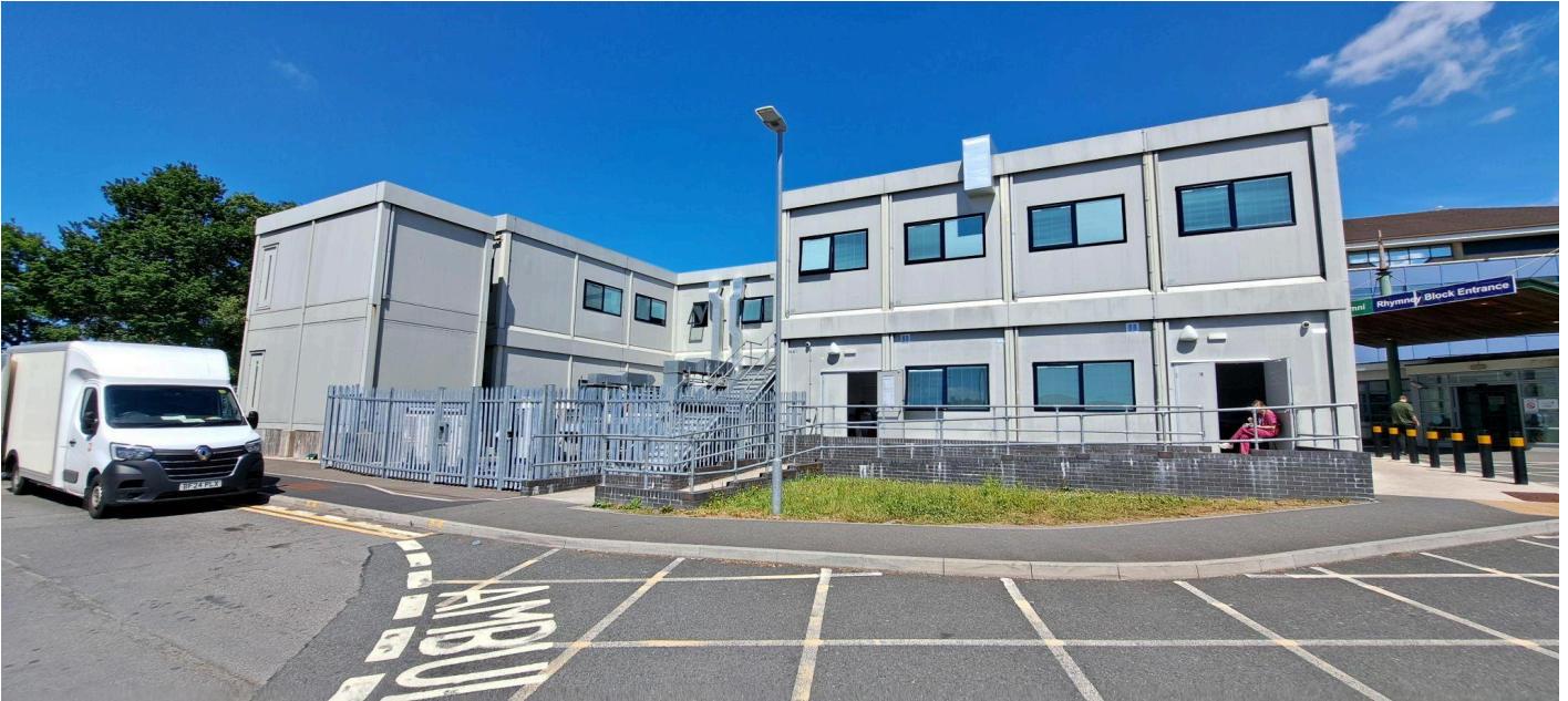
Unit 2 view from north
