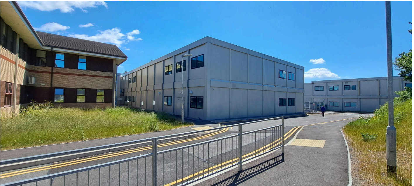
Unit 2 view from south-east
