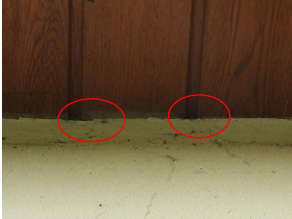
Photo 9: Example of Gaps Between External Wall and Door Frame
