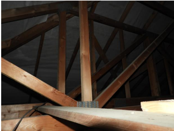
Photo 11: Loft Void with Breathable Membrane
