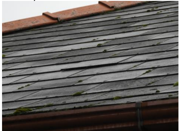
Photo 6: Example of Raised Slates (Southern Elevation)
