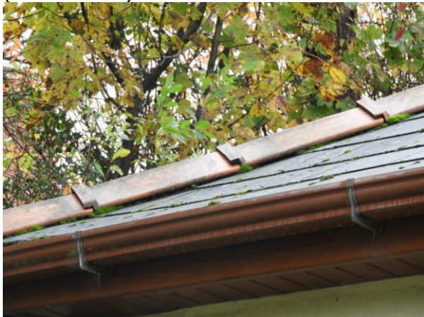
Photo 5: Example of Gaps Beneath Ridge Tiles (Southern Side)
