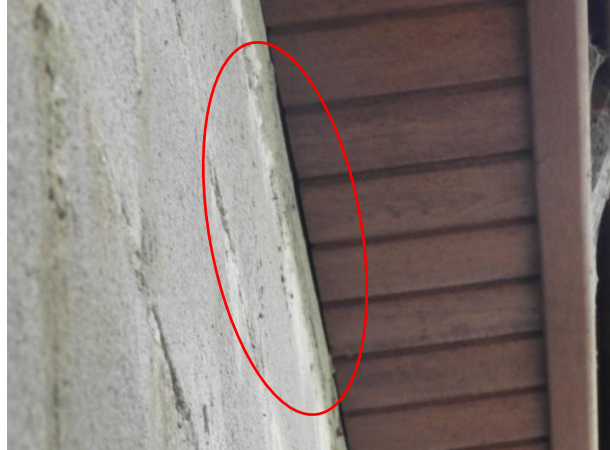
Photo 10: Gap Above Roller Shutter Door
