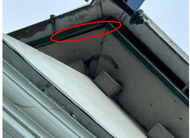
Photo 18: Lifted Lead Flashing North-Eastern Elevation (Circled)
