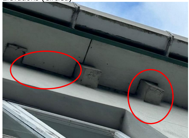
Photo 12: Example of Gaps Between Soffit Box and External Wall and Gaps Around Rafters on All Elevations (Circled)
