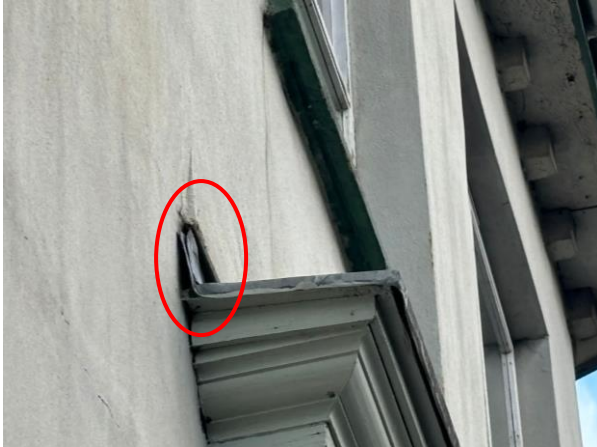
Photo 15: Gap Between Decorative Timber and External Wall on the Eastern Elevation (Circled)
