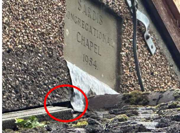
Photo 6: Raised Lead Flashing on the Northern Gable End (Circled)
