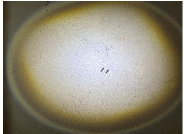
Photo 22: Example of Bat Dropping on Interior Wall
