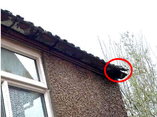
Photo 5: Loosely Fitted Tile on the Western Pitch of Chapel Roof (Circled)
