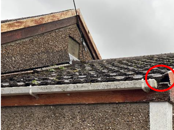
Photo 5: Loosely Fitted Tile on the Western Pitch of Chapel Roof (Circled)
