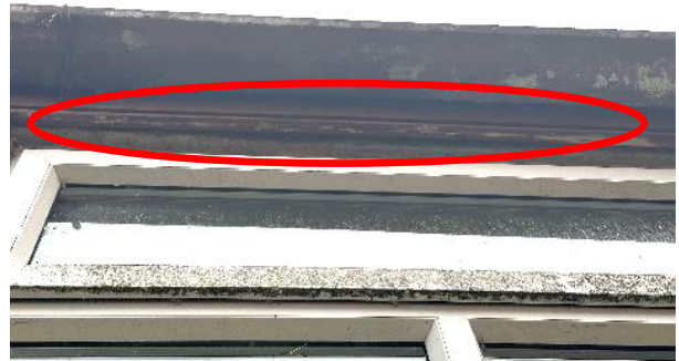
Photo 16: Gap Present at the Apex of the Interior Wall on the Southern Elevation
