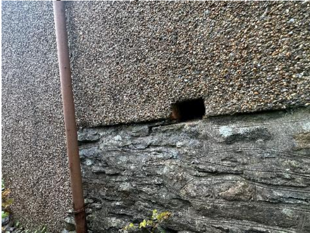
Photo 11: Exposed Stone Underneath the Rendering with Missing Brick
