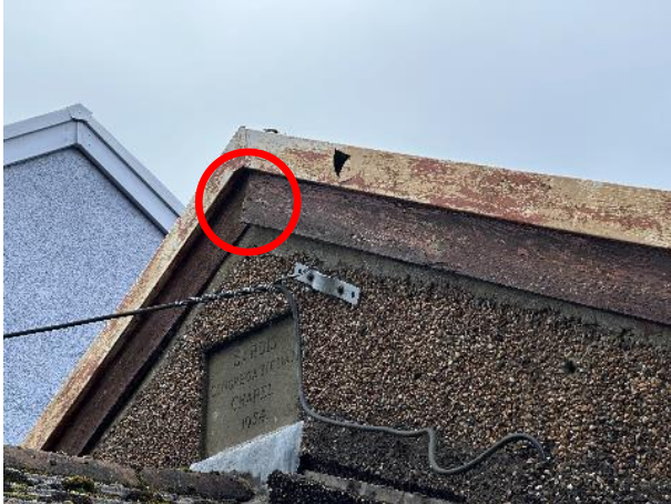
Photo 9: Gaps on the Metal Vent on the Eastern Side
