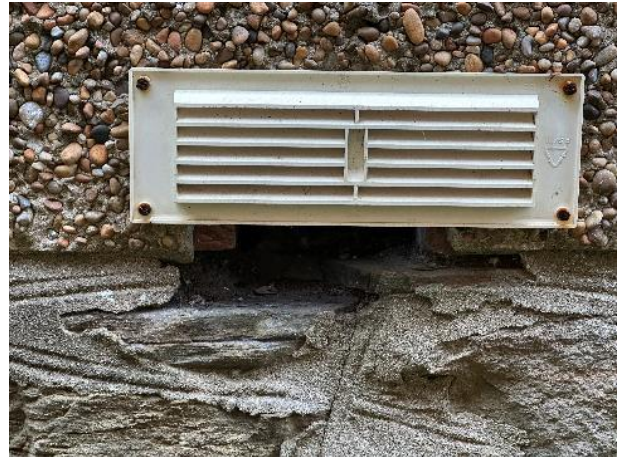
Photo 12: Missing Brick Underneath the Rendering
