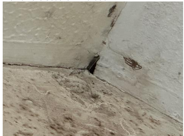
Photo 18: Window Tightly Sealed to the Frame. Large Gap Present Between the Window Frame and the Fascia
