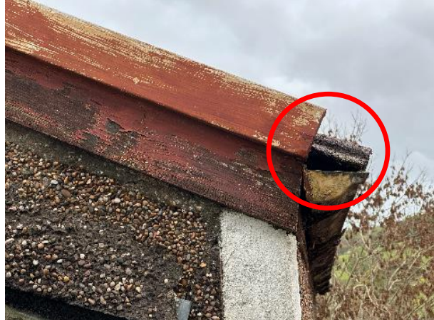
Photo 6: Raised Lead Flashing on the Northern Gable End (Circled)
