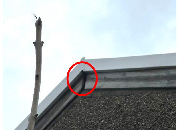
Photo 10: Gaps Underneath the uPVC Vent on the Western Side
