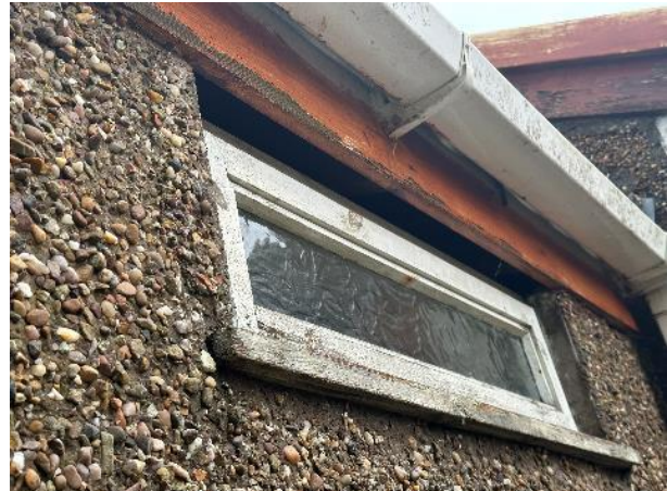
Photo 18: Window Tightly Sealed to the Frame. Large Gap Present Between the Window Frame and the Fascia
