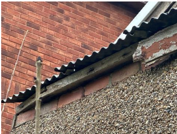
Photo 17: Gaps Between the Corrugated Sheeting and the Timber Support on Easternmost Extension. Fascia is in Poor Condition
