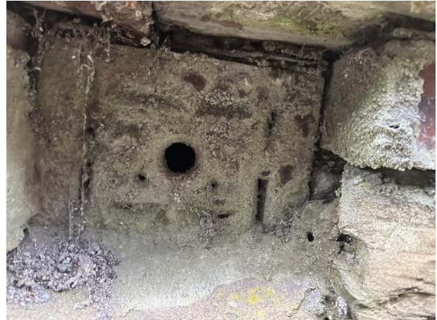
Photo 12: Missing Brick Underneath the Rendering
