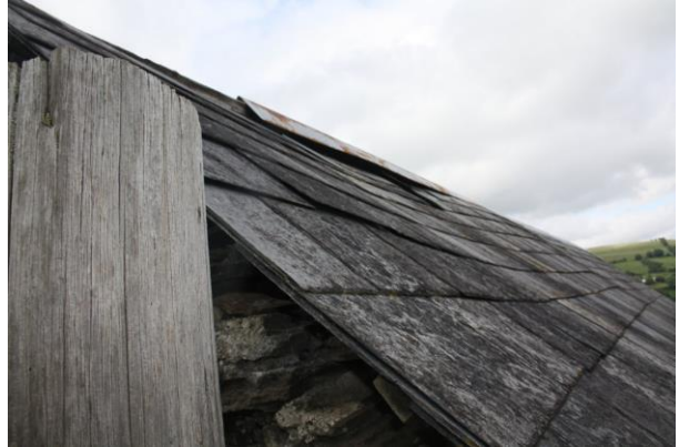
Photo 8: Gap under ridge at eastern gable end
