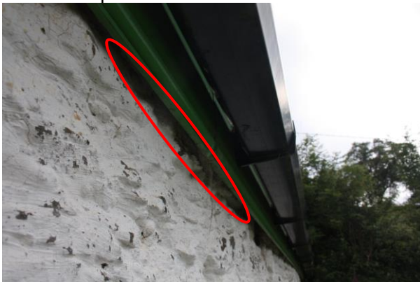
Photo 9: Example of crevices in external stonework
