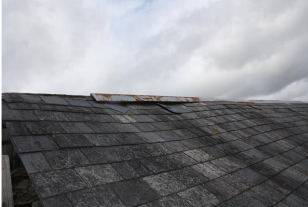
Photo 7: Gaps under fascia on northern elevation
