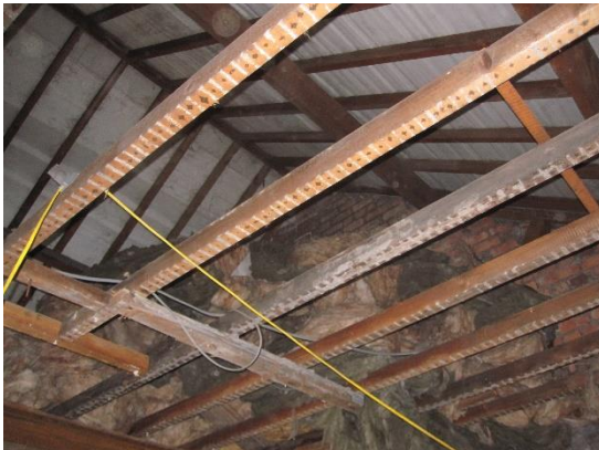
Plate 7: Main loft area, illustrating absence of ceilings and fitment of breathable membrane
