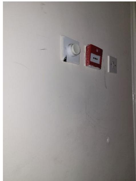
There is no documentation evident to verify that regular inspection and testing of the Fire Alarm System occurs.
