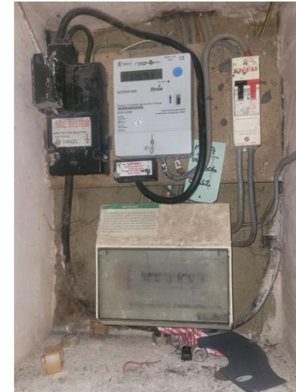
The consumer unit is of the insulated type fitted with a 30milliamp Double Pole RCD Main Switch which provides additional earth fault protection which is required for all lighting circuits in a domestic type dwelling and socket outlet circuits rated at 32 amp or less. Miniature Circuit Breakers provide individual circuit protection against overload and short circuit faults between live conductors.
