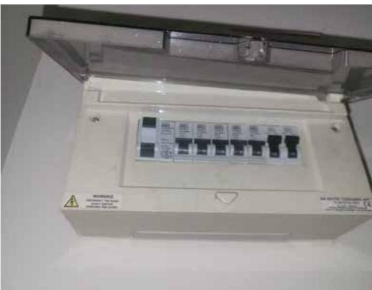
The consumer units are of the insulated type fitted with a 30milliamp Double Pole RCD Main Switch which provides additional earth fault protection which is required for all lighting circuits in a domestic type dwelling and socket outlet circuits rated at 32 amp or less. Miniature Circuit Breakers provide individual circuit protection against overload and short circuit faults between live conductors.
