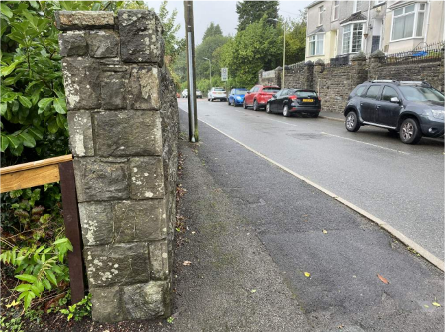
Existing site access View West
