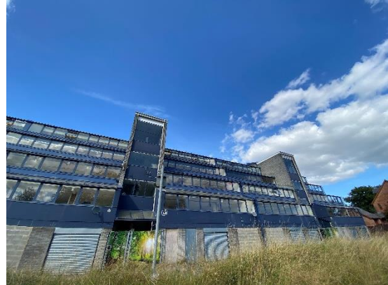
Plate 2: Southern elevation of the Lower Building
