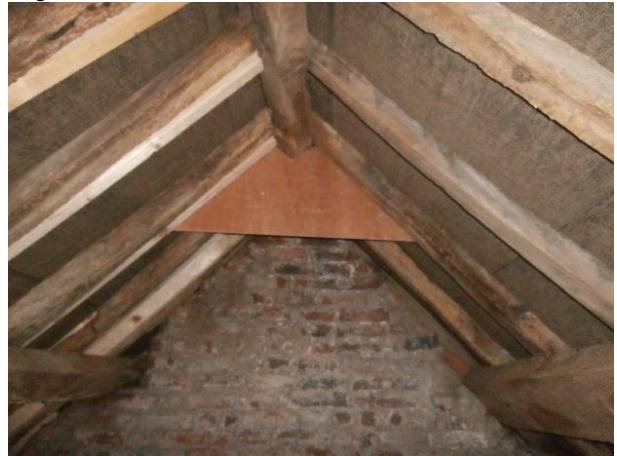
Figure 8: Baffle enhancement feature
