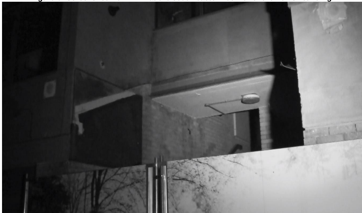
Figure 6: Screenshot from NVA at the south-eastern corner of the Lower building
