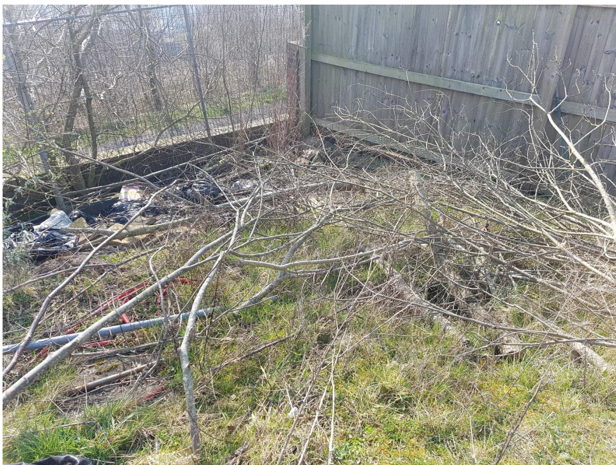
Photo 2 Corner of the plot showing the retaining wall on Twynygarreg
