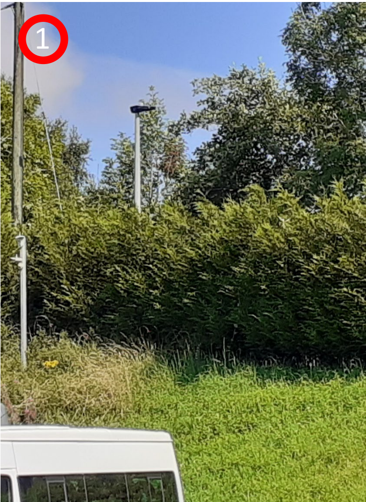
Existing lighting columns along pedestrian footpath
