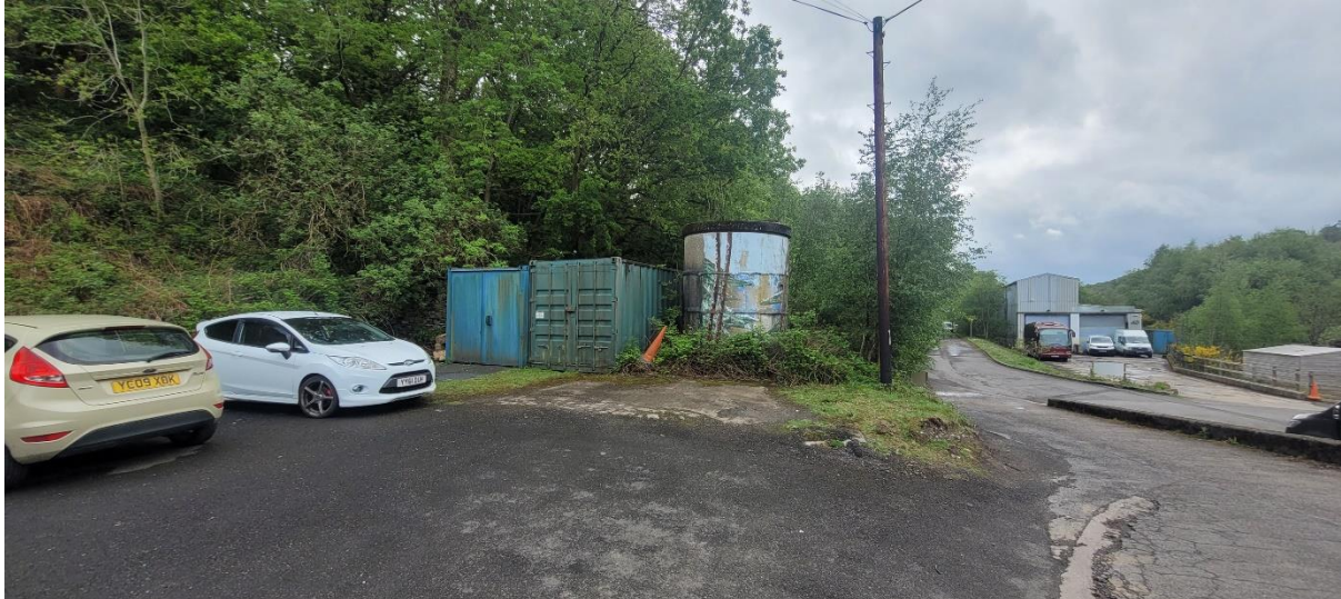
Plate 2 – Entrance (looking south)
