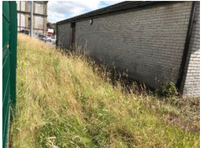
Northern boundary of site looking east
