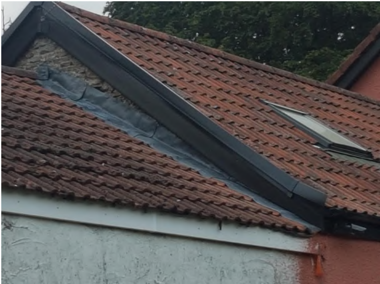
2) Gable end of family room section
