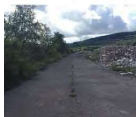
Tarmac road along north east looking south
