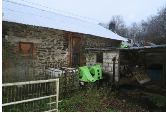
PART OF EAST ELEVATION WITH LOWER (CATTLE) BARN:
