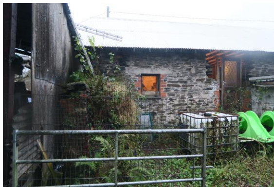
PART OF EAST ELEVATION: NOTE WALL TO SIDES OF DOOR – DOOR JAMBS TO BE REBUILT AND BONDED INTO EXISTING:
