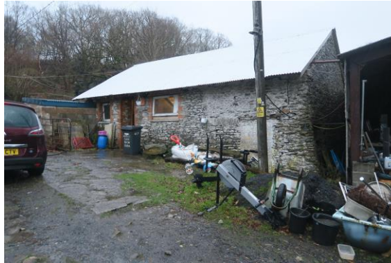
EAST ELEVATION: NOTE BRICK SURROUND TO OPENINGS AND INFILLED OPENINGS AT SOUTH END:
