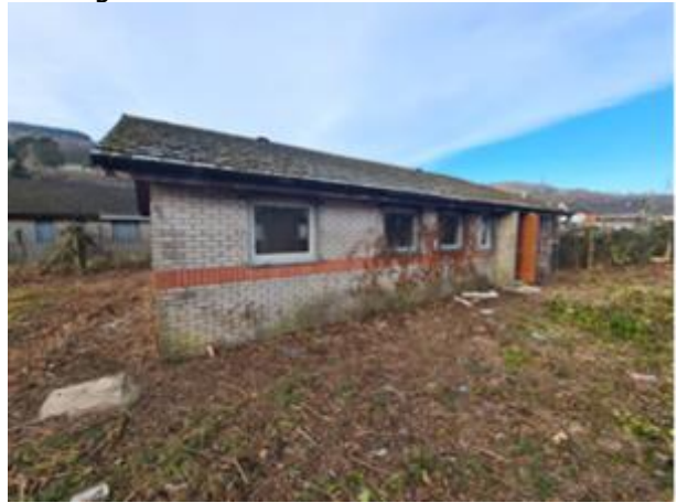
Photo 2: Eastern Elevation of Former Surgery Building
