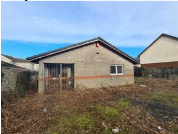
Photo 1: Southern Elevation of Former Surgery Building
