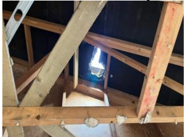
Photo 18: Tear in Bitumen Felt Roof Lining
