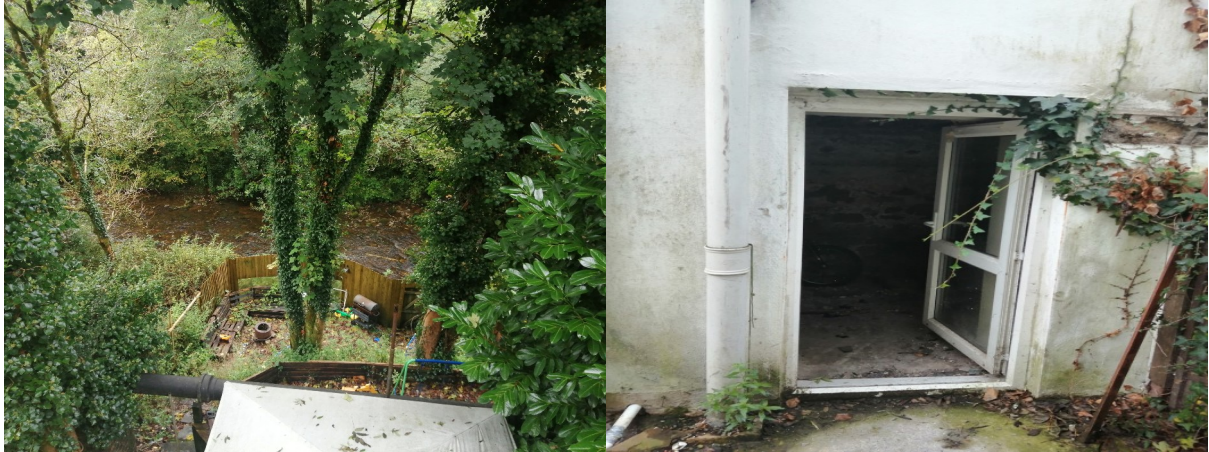
Access to ground floor storage areas at rear
