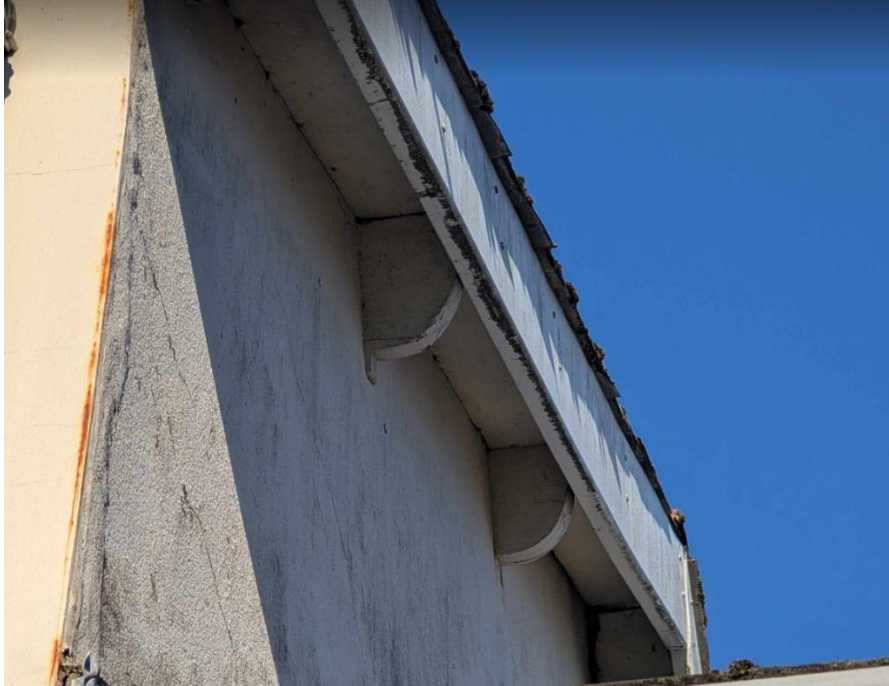
Plate 2-sealed eaves at front of property
