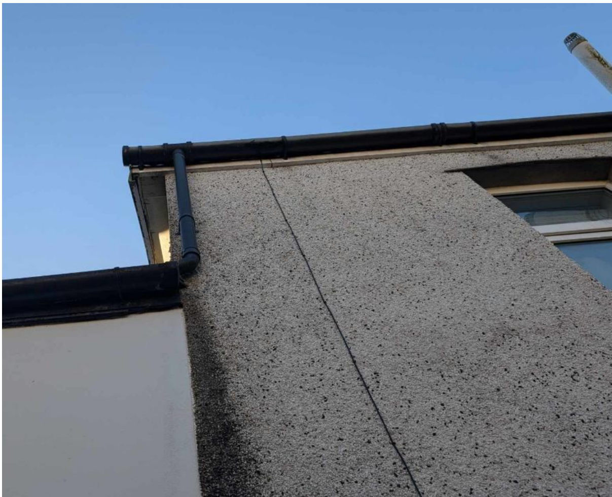
Plate 4-sealed fascia at rear of property
