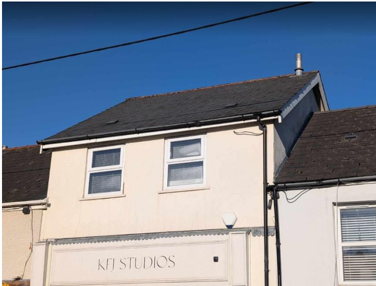
Plate 4-sealed fascia at rear of property
