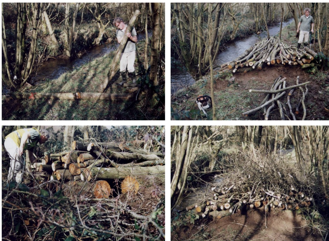
Figure MP6 Construction of Habitat Pile
