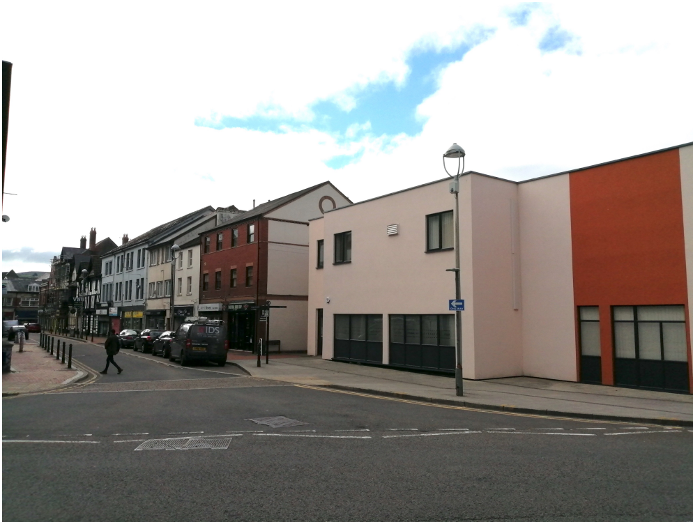
GLEBELAND STREET GENERAL VIEW
