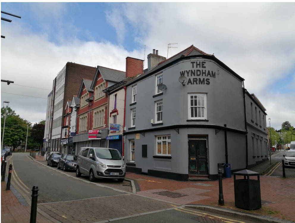
GLEBELAND STREET GENERAL VIEW
