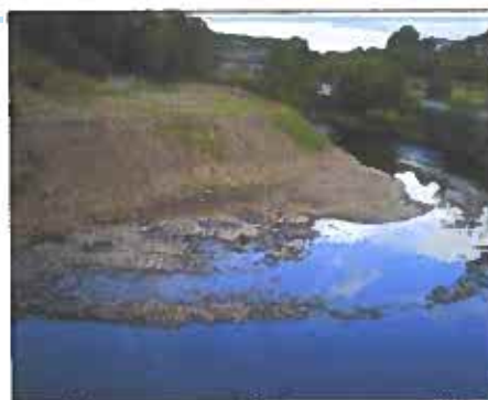
30/09/2009 – Looking upstream from footbridge
