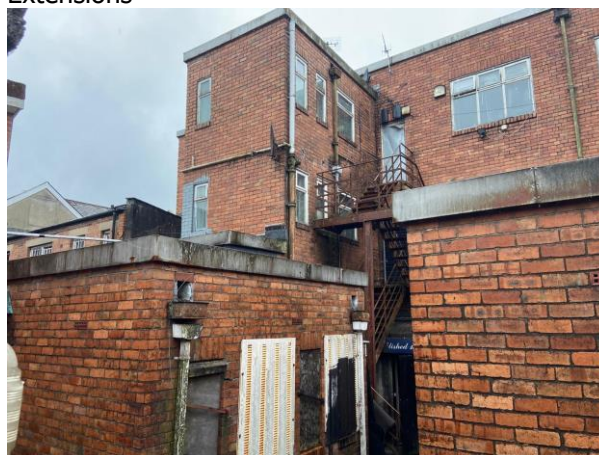
Photo 2: Eastern Rear Showing Single-storey Extensions
