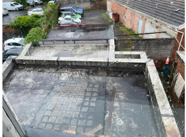
Photo 6: Easternmost Single-storey Extension Showing Vent Bitumen Felt Roof
