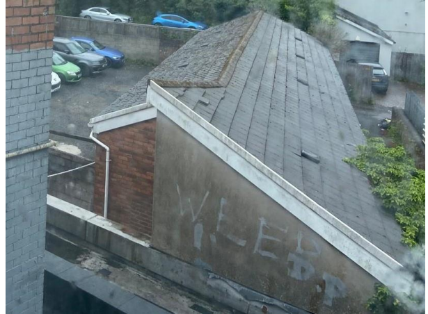
Photo 17: Western Elevation and View of the Roof
