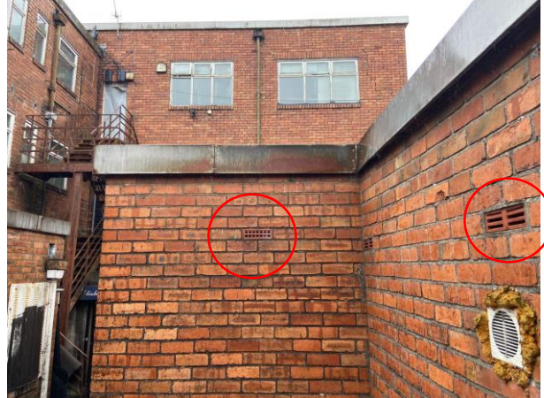
Photo 8: Example of Vents on the Single-storey Extensions
