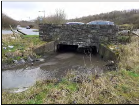
7. Photo of bridge
