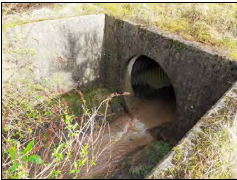
1. Photo showing culvert
