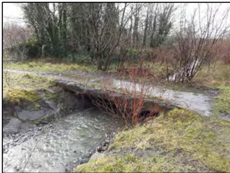
8. Photo of bridge
