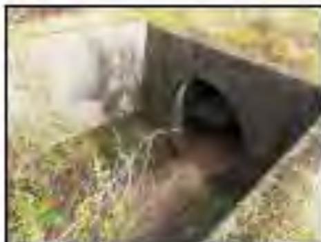
1. Photo culvert pipe
