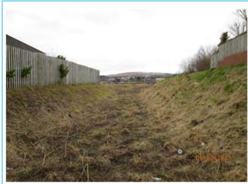
Figure 4 - Looking downstream immediately downstream of the road culvert in Bradley Gardens
