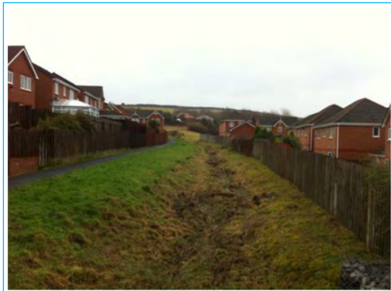
Figure 5 - Looking upstream in the Bradley Gardens catchment watercourse at the smallest flow capacity cross section
