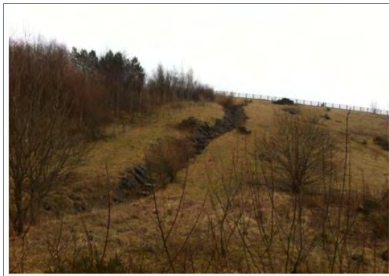
Figure 3 - Engineered channel immediately downstream of the Morlais B outfall
