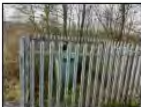
2. Photo steel security point
